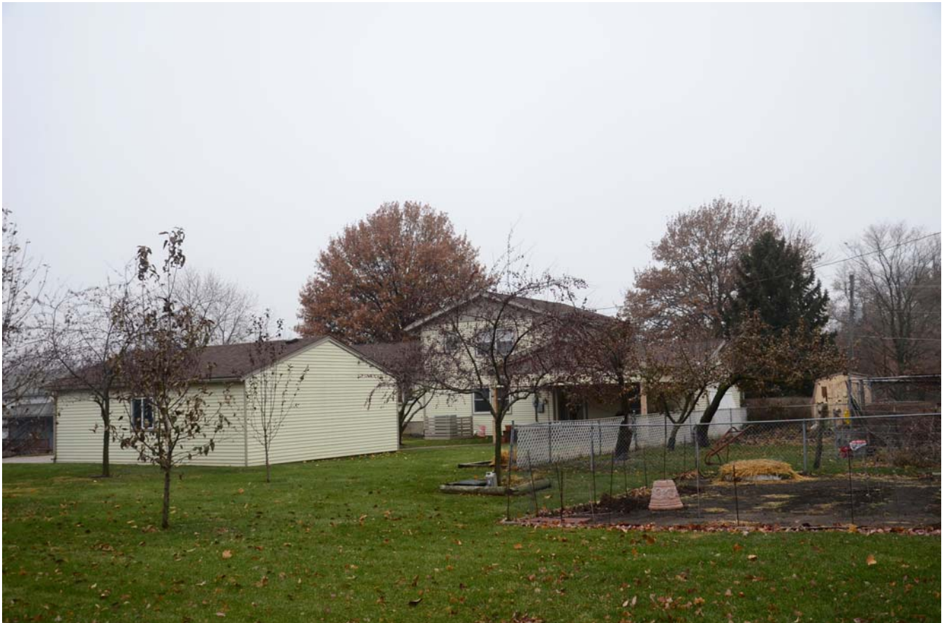
Photograph 92-00750-004 - Garage, looking southeast (December 2014)
