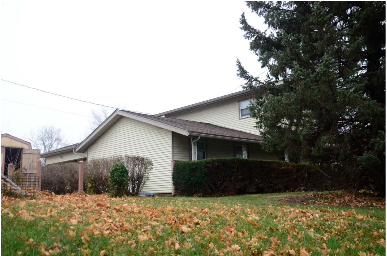
Photograph 92-00750-003 - House, looking southeast (December 2014)
