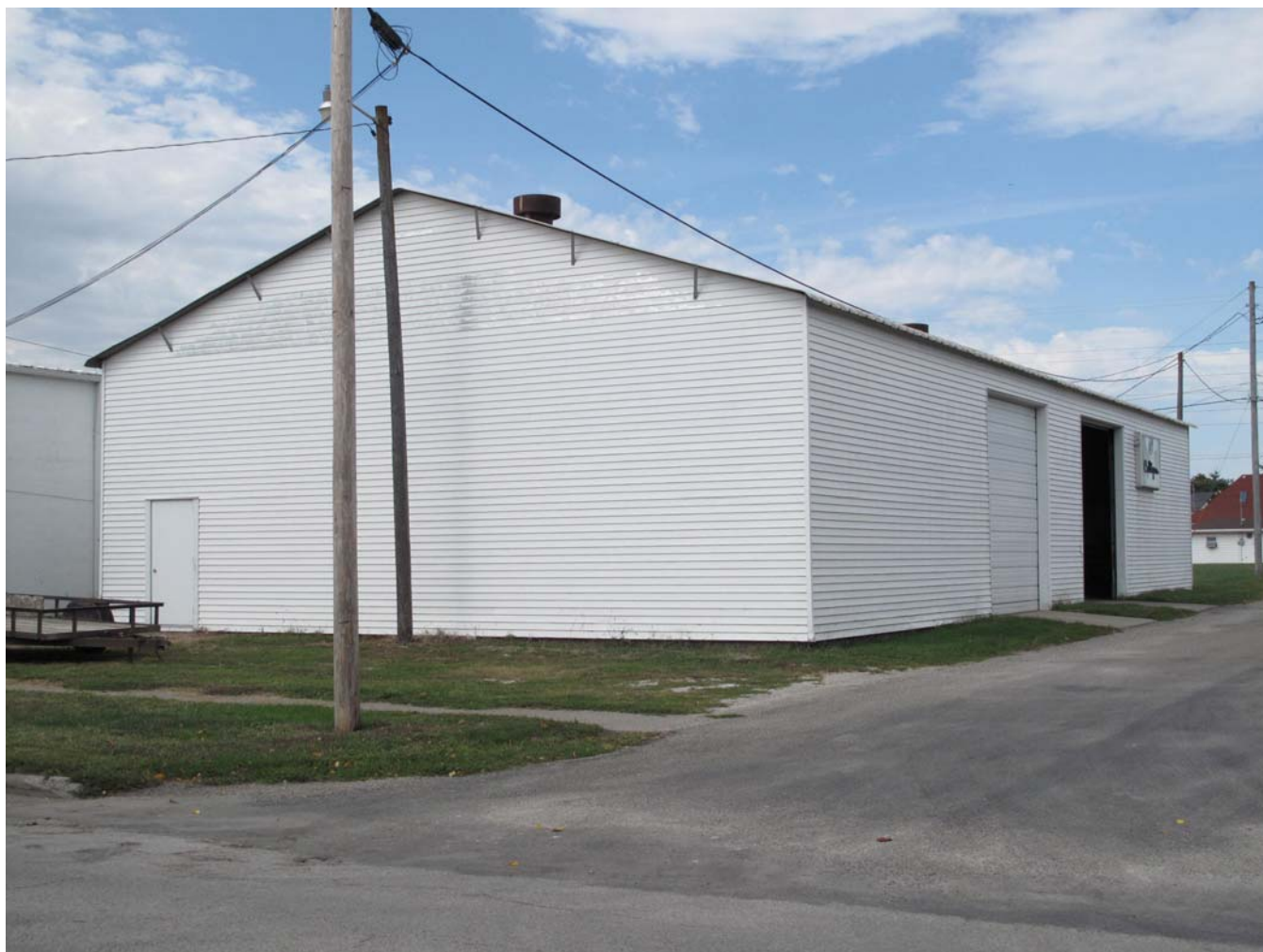
Photograph 92-00589-001 - South and east elevations, looking northwest (McCarley, September 20, 2011)
