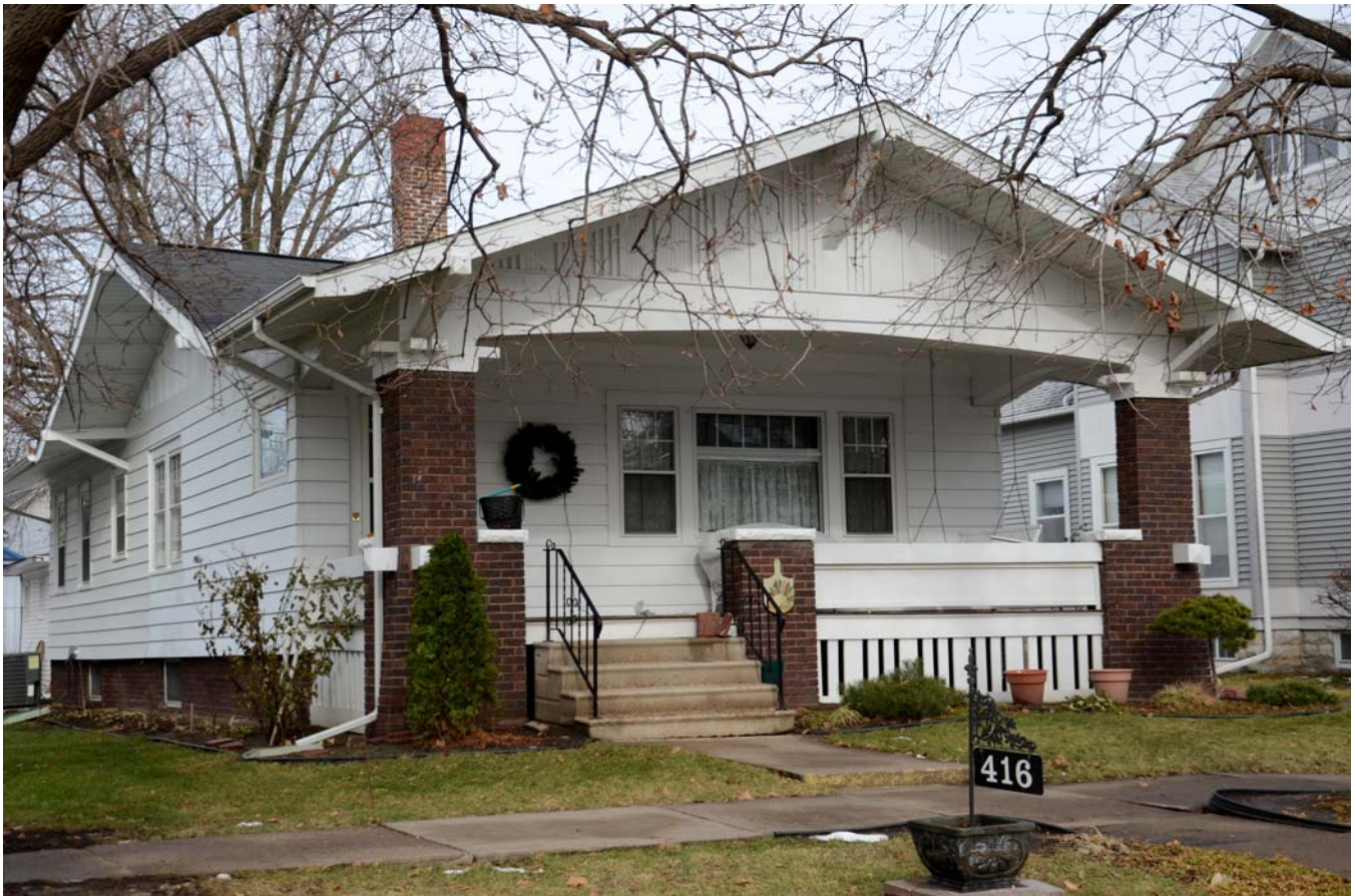
Photograph 92-00387-001 - House, looking northeast (December 2014)
