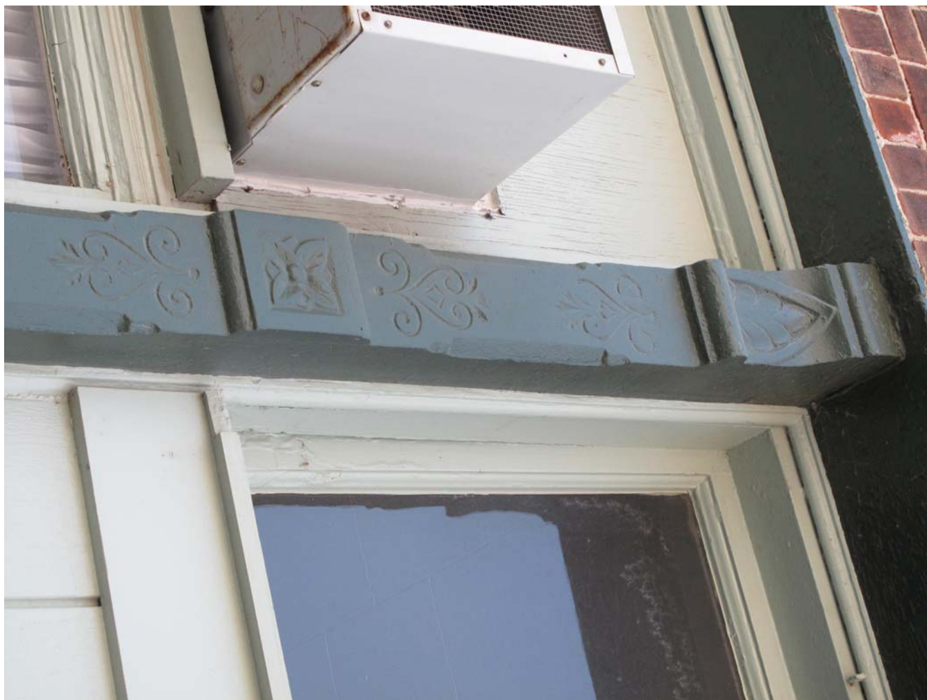
Photograph 92-00545-008 - Column detail on 217 storefront, looking southeast (McCarley, September 20, 2011).
