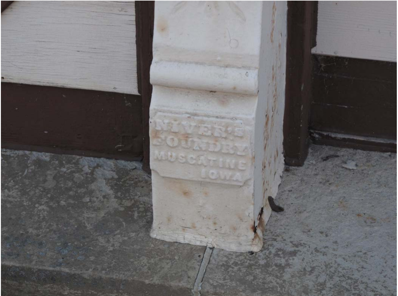
Photograph 92-00545-005 - Column detail on 213 storefront, looking south (McCarley, September 20, 2011).
