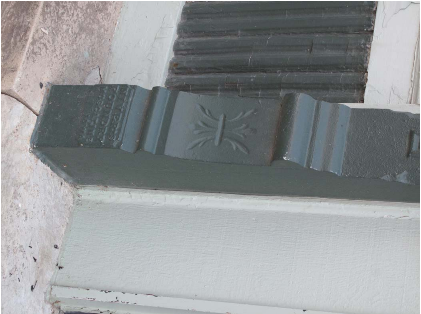
Photograph 92-00545-007 - Column detail on 217 storefront, looking southeast (McCarley, September 20, 2011).
