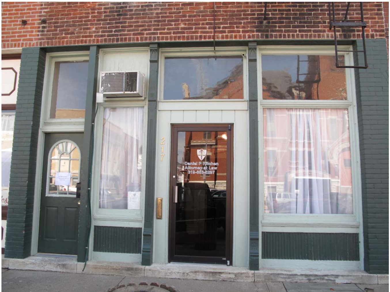
Photograph 92-00545-006 - 217 storefront, looking south (McCarley, September 20, 2011).
