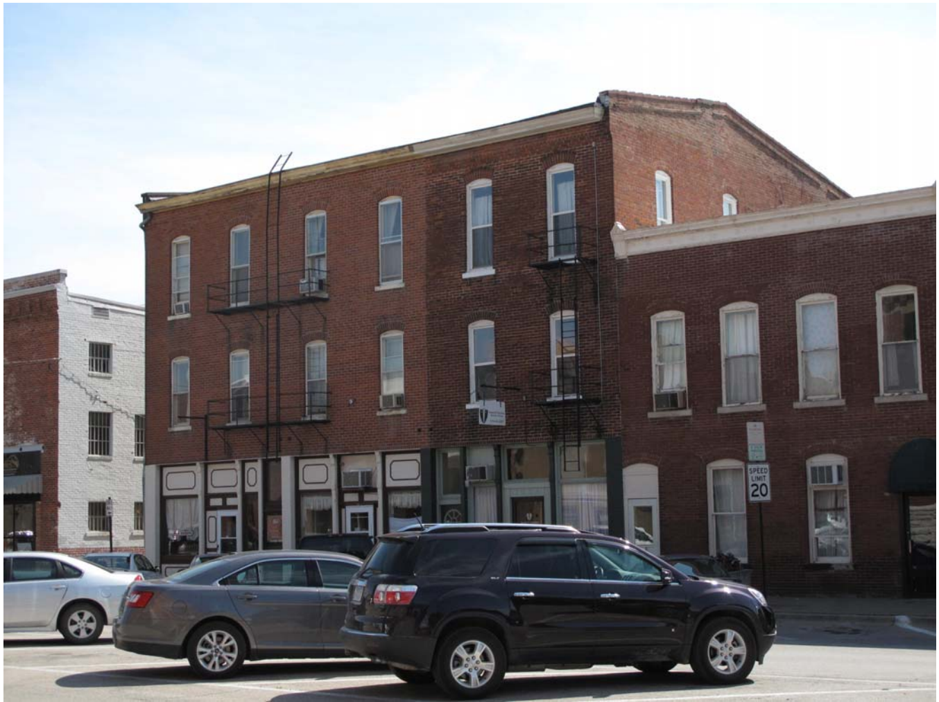
Photograph 92-00545-002 - Front (north) and west elevations, looking southeast (McCarley, September 20, 2011).
