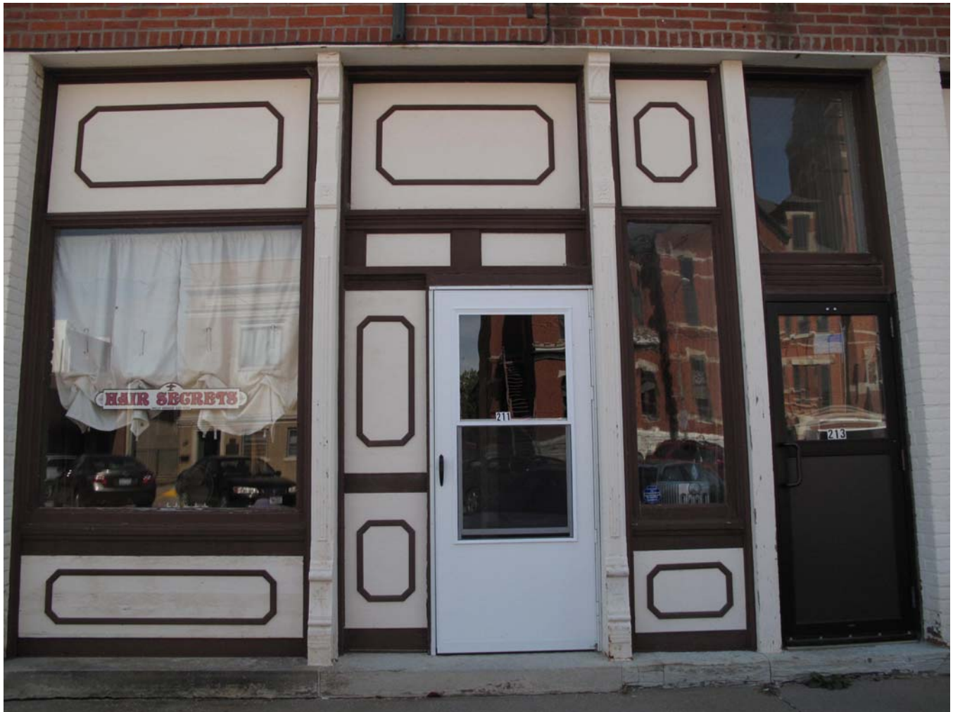
Photograph 92-00545-004 - 213 storefront, looking south (McCarley, September 20, 2011).
