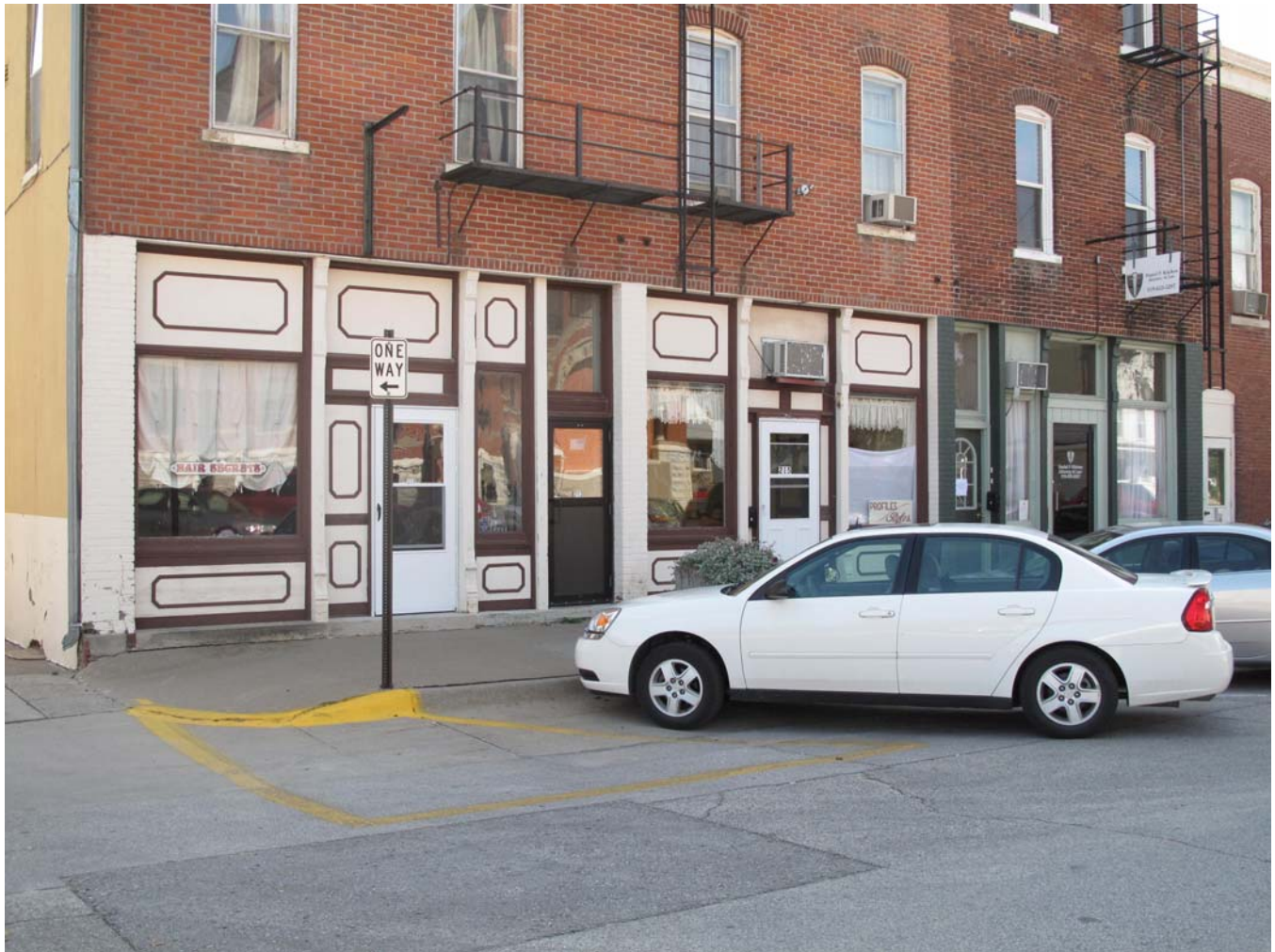
Photograph 92-00545-003 - Storefronts, looking southwest (McCarley, September 20, 2011).
