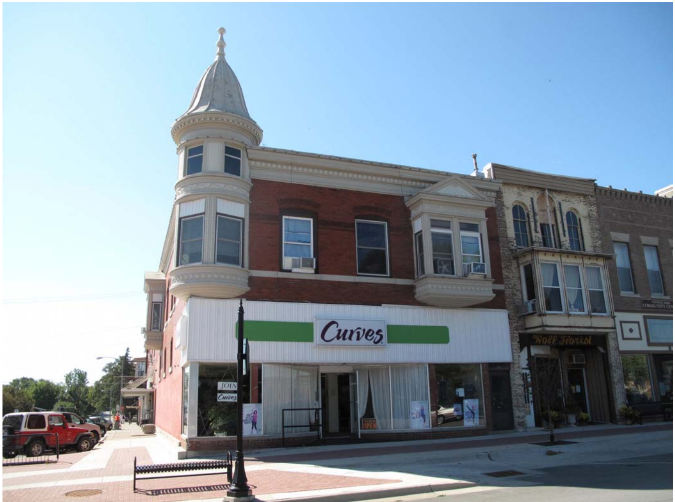
Photograph 92-00601-002 - North side, looking south (McCarley, September 20, 2011)
