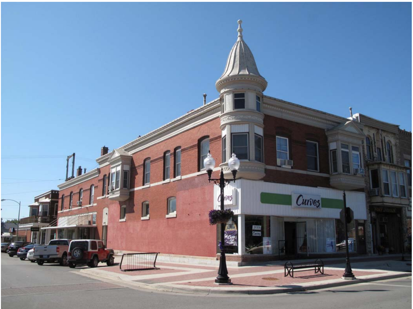
Photograph 92-00601-001 - East and north sides, looking southwest (McCarley, September 20, 2011)
