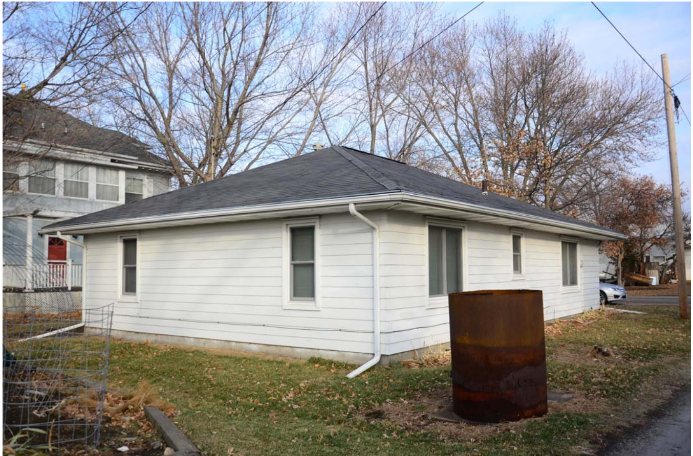
Photograph 92-00759-002 - House, looking northeast (December 2014)
