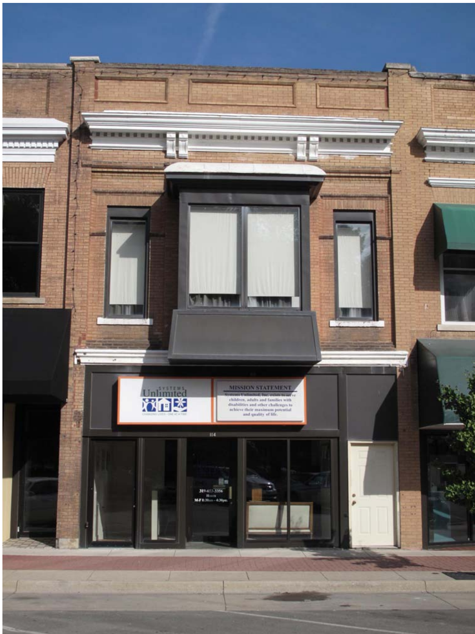
Photograph 92-00514-001 - West elevation, looking east (McCarley, September 20, 2012)
