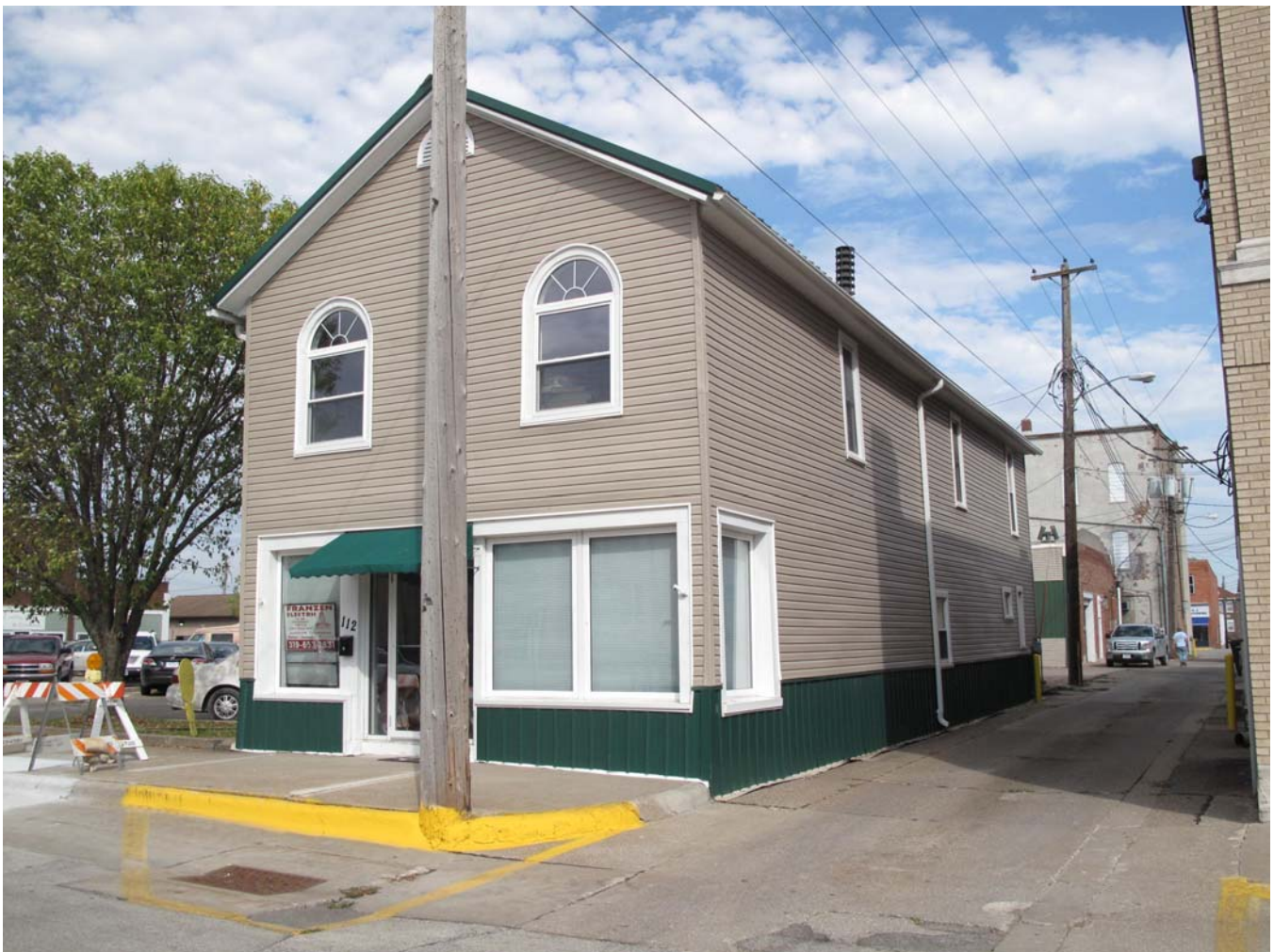
Photograph 92-00552-001 - West and south elevations, looking northeast (McCarley, September 20, 2011)
