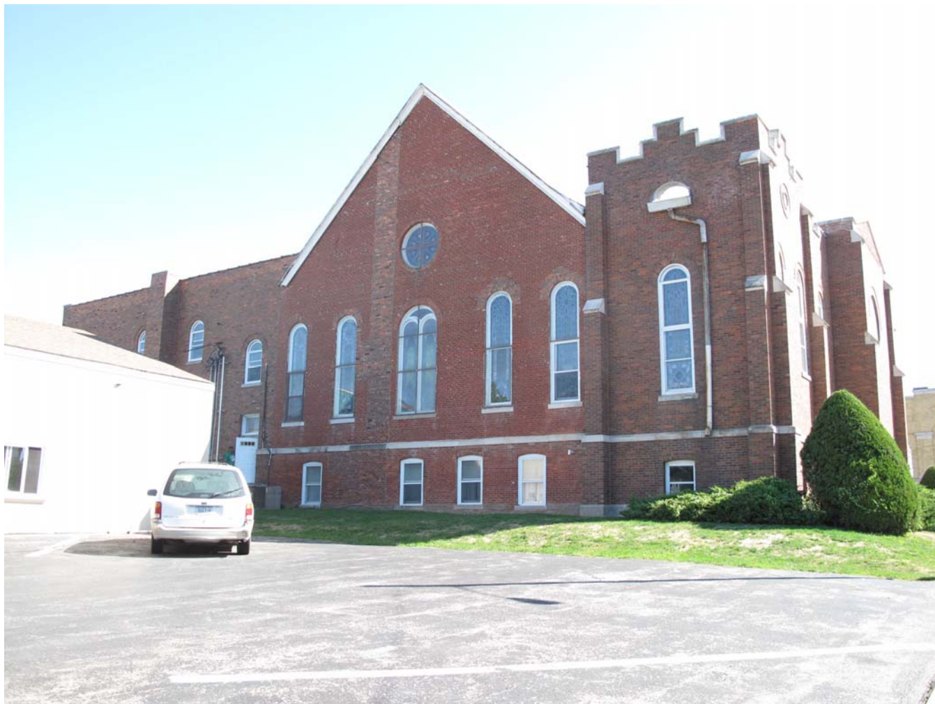
Photograph 92-00572-005 - West elevation, looking east (McCarley, September 20, 2011)
