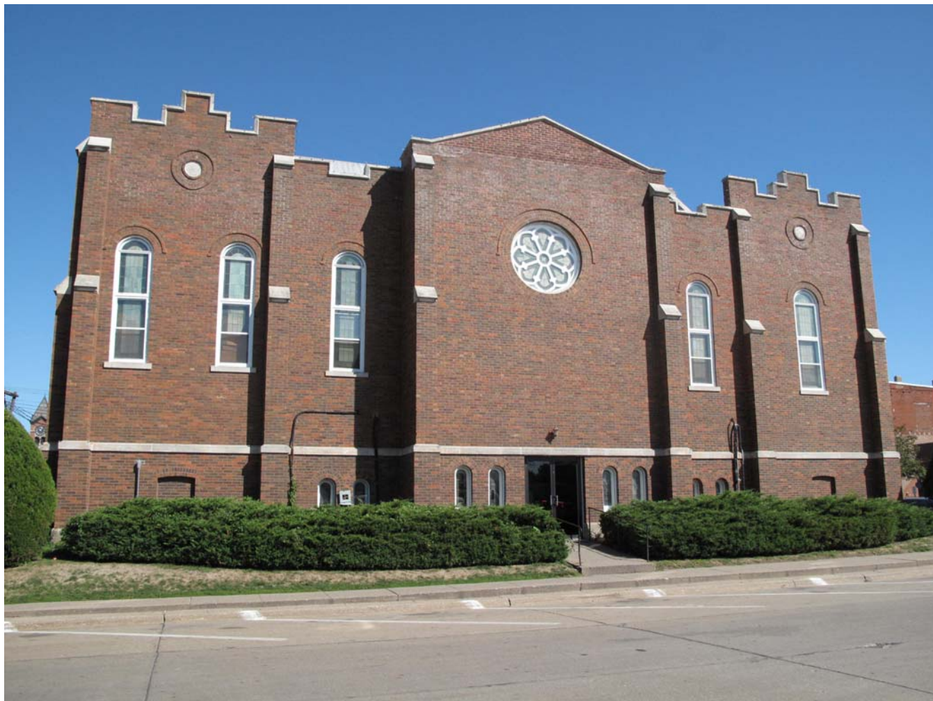
Photograph 92-00572-004 - South elevation, looking north (McCarley, September 20, 2011)
