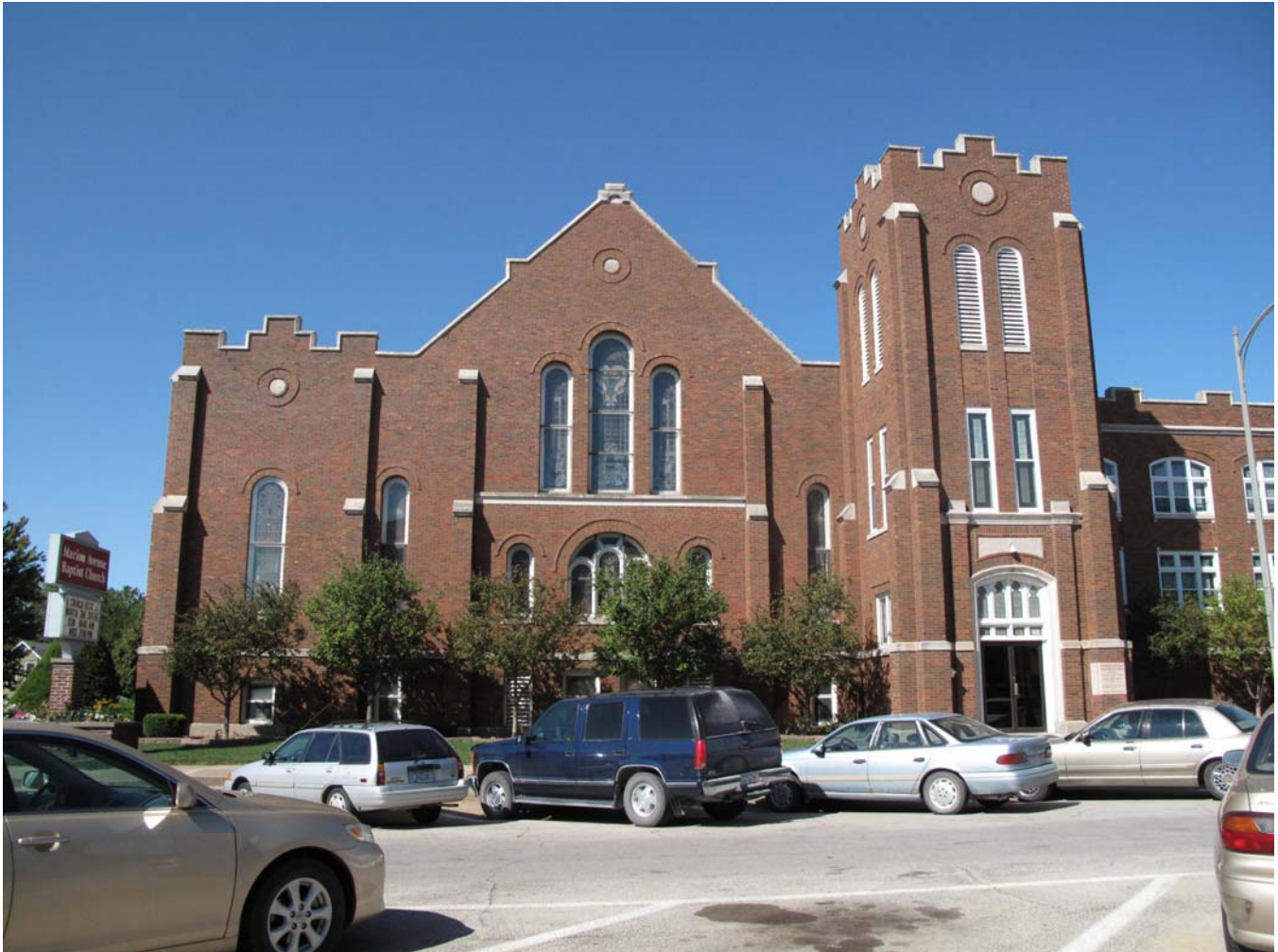
Photograph 92-00572-002 - East elevation, looking west (McCarley, September 20, 2011)
