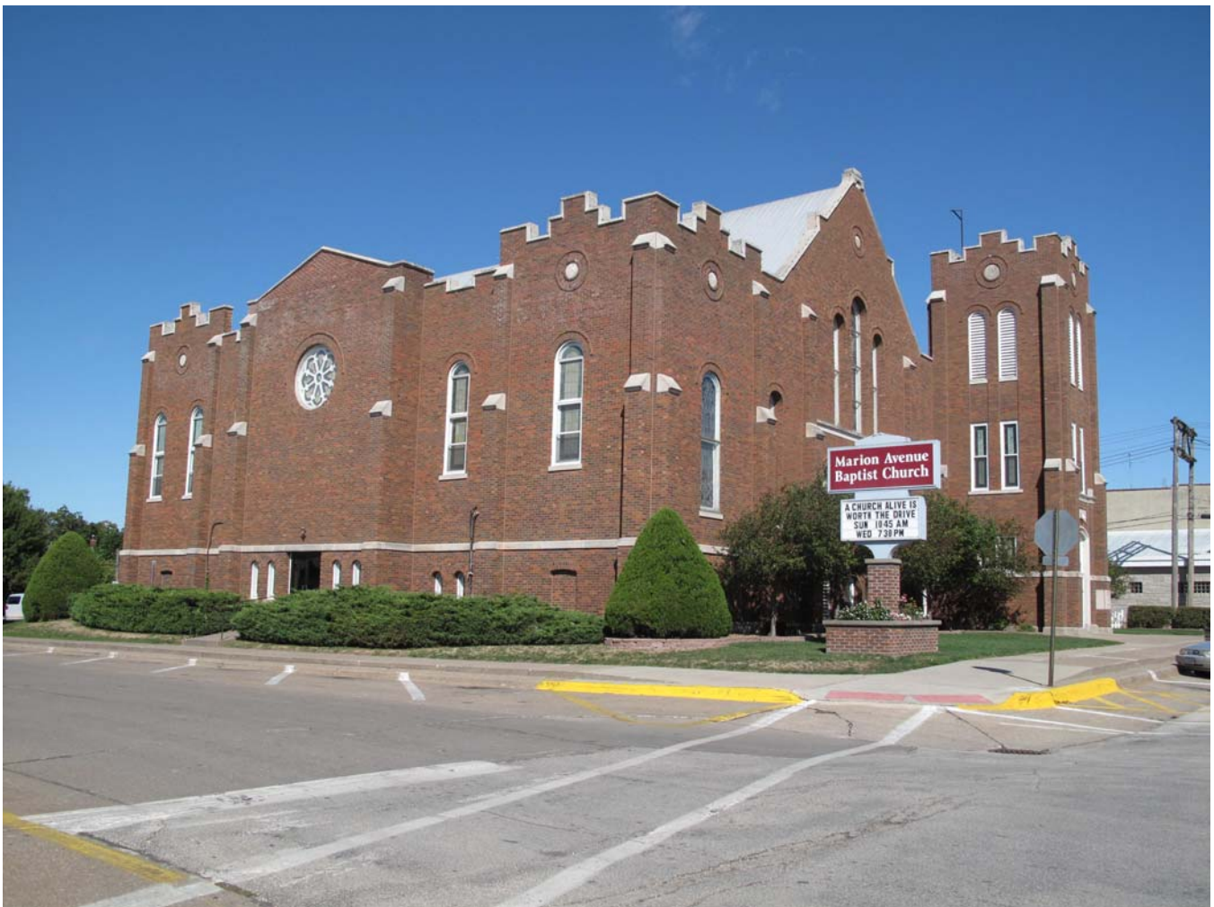
Photograph 92-00572-001 - South and east elevations, looking northwest (McCarley, September 20, 2011)
