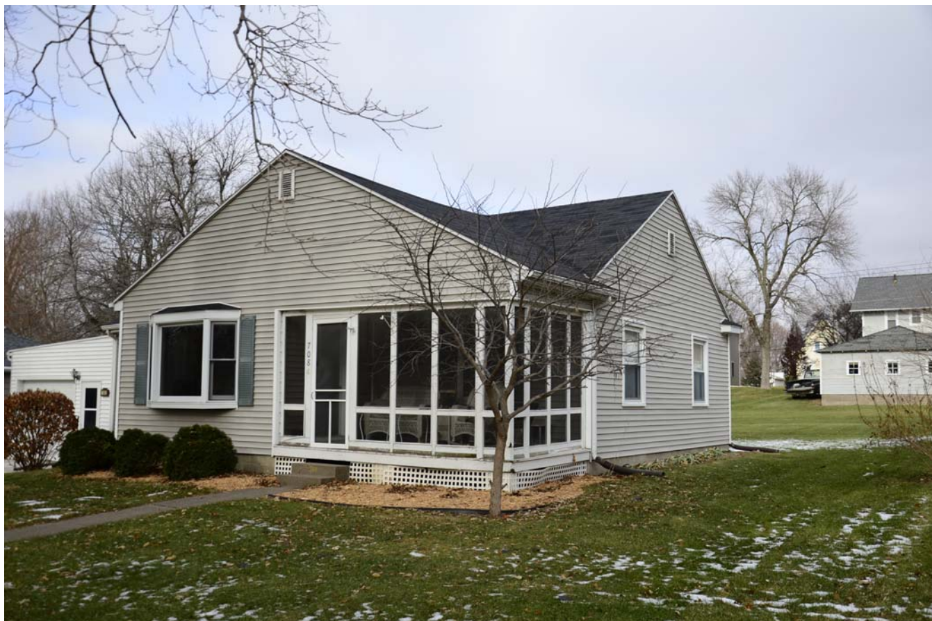
Photograph 92-00767-002 - House, looking northwest (December 2014)
