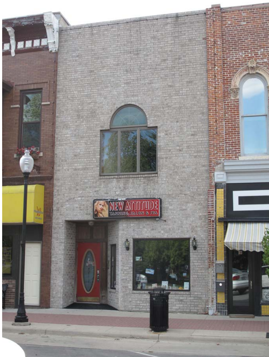
Photograph 92-00559-001 - East elevation, looking west (McCarley, September 20, 2011)
