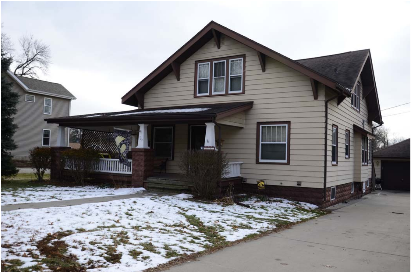
Photograph 92-00790-001 - House, looking southeast (December 2014)
