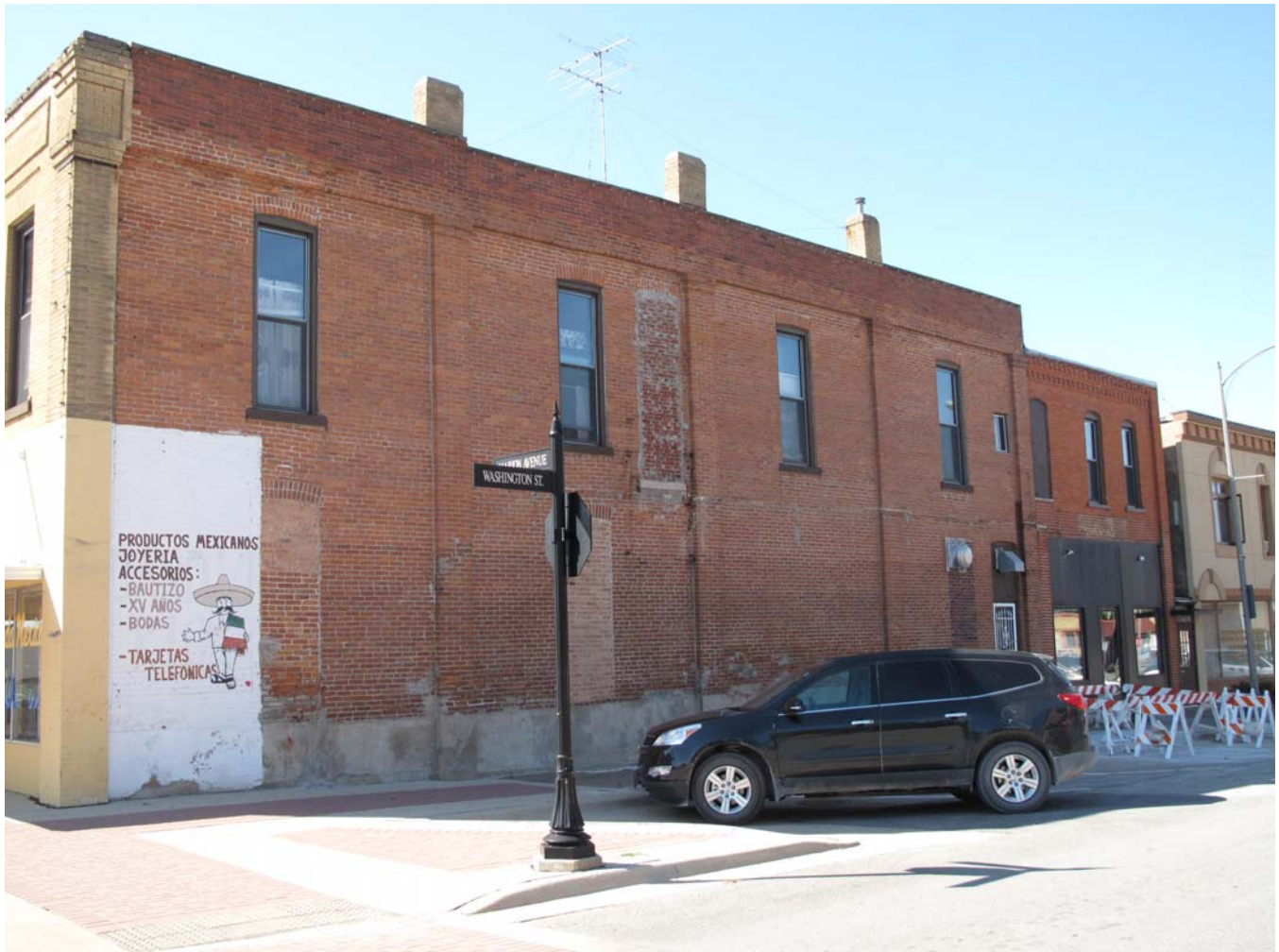
Photograph 92-00566-002 - North elevation, looking southwest (McCarley, September 20, 2011)
