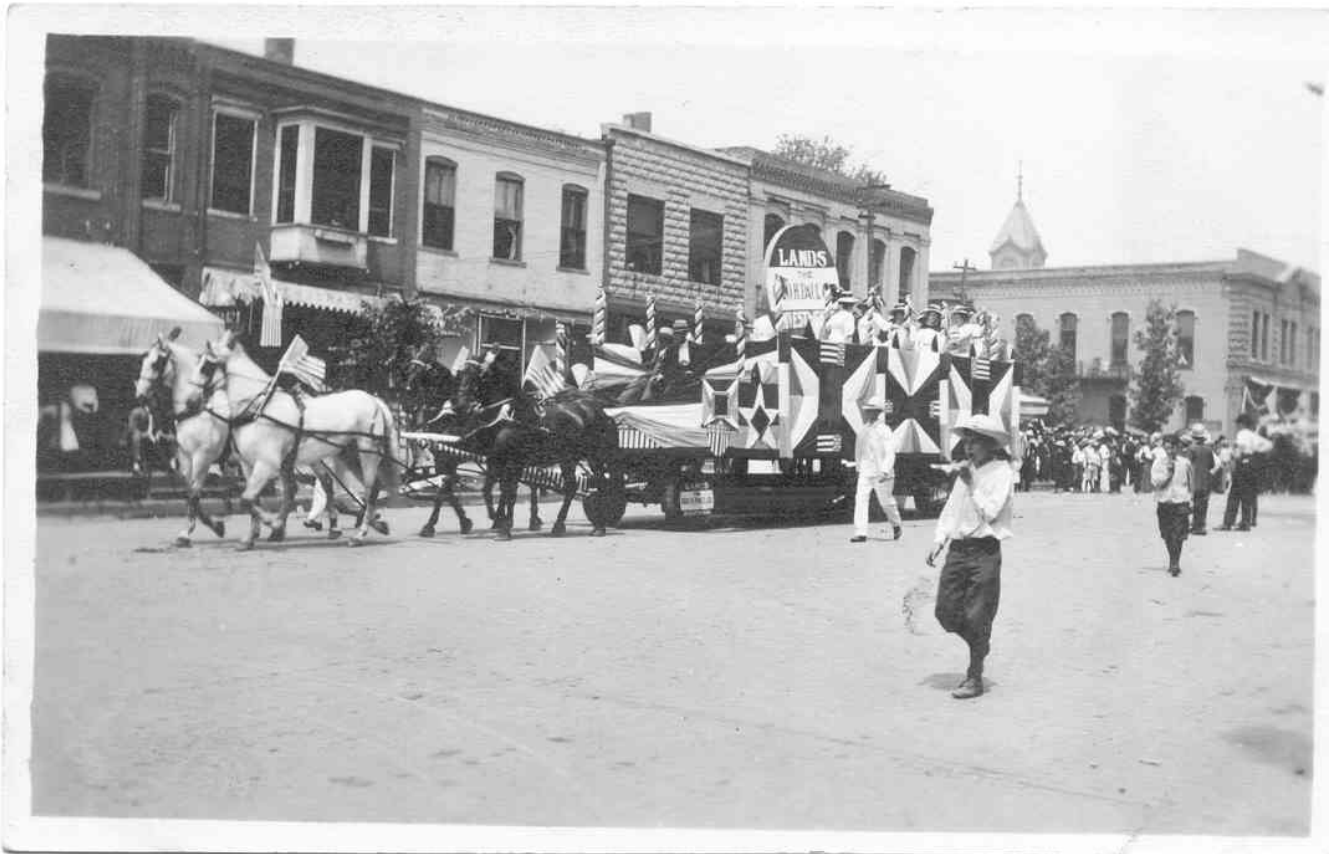
200 block of S. Marion, looking northwest, after c.1910 rusticated concrete block façade applied to 205 S. Marion, before c.1912 remodel of corner grocery building (Patterson collection)
