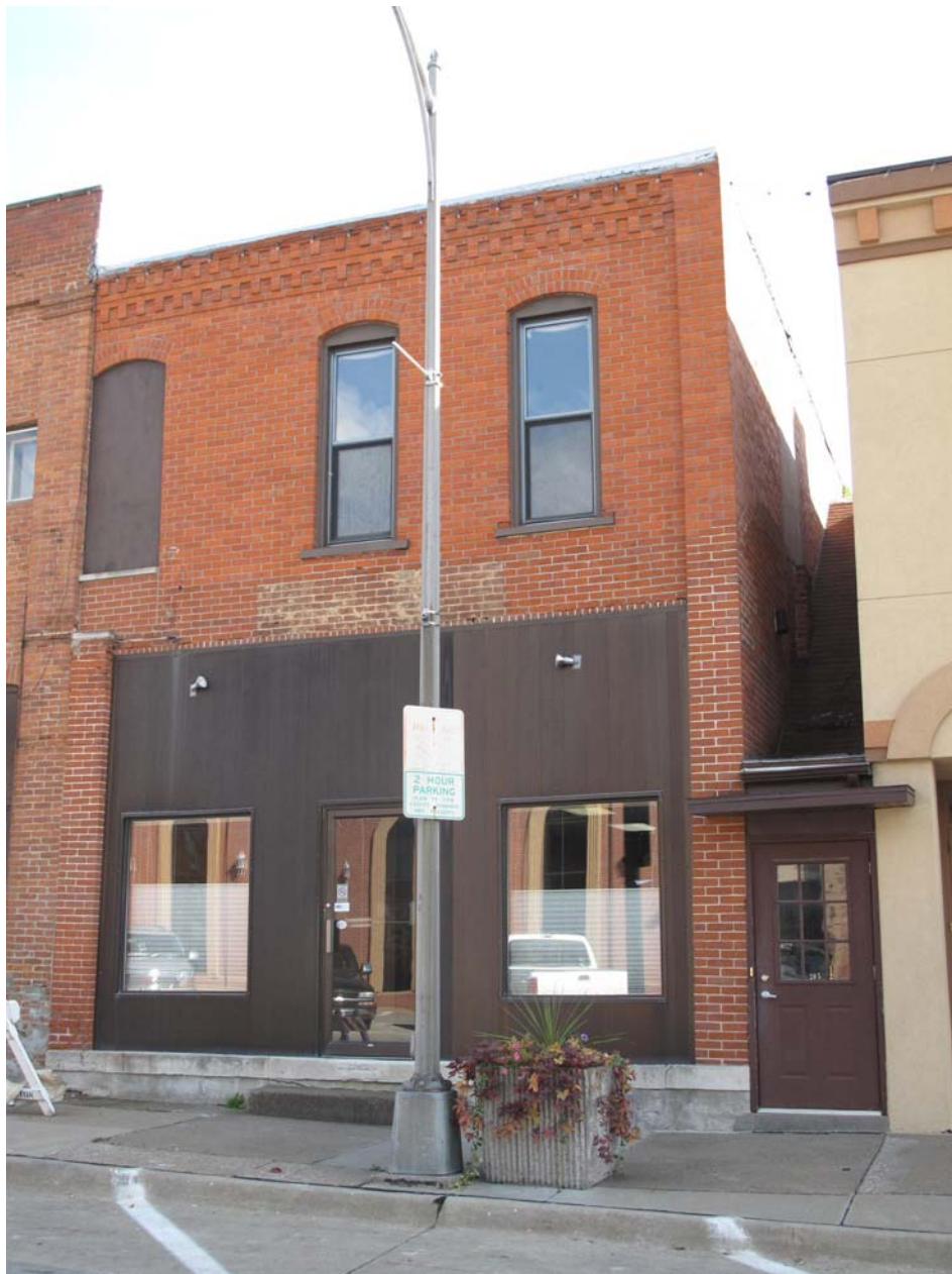
Photograph 92-00566-003 - North elevation, looking south (McCarley, September 20, 2011)
