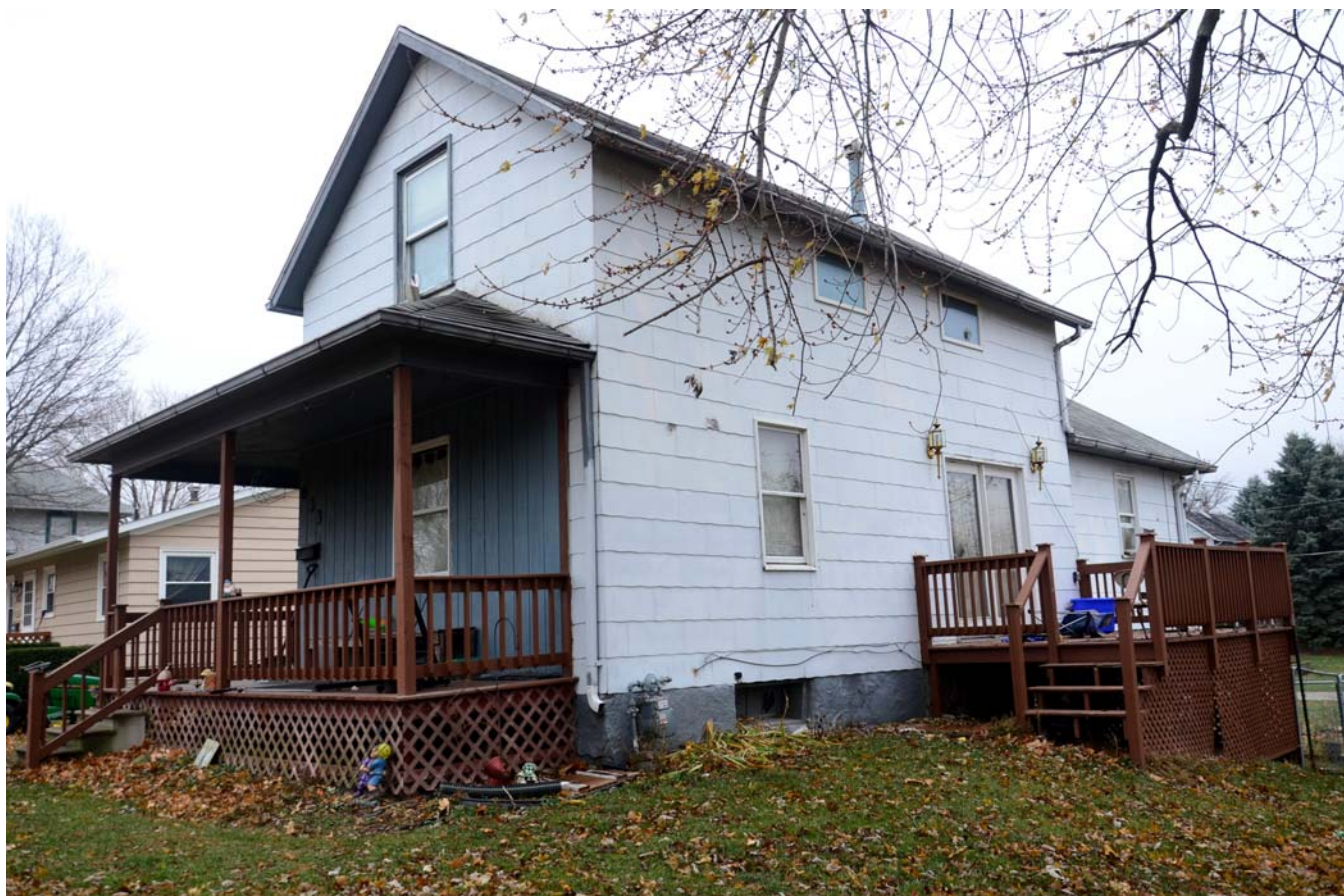
Photograph 92-00756-002 - House, looking southeast (December 2014)
