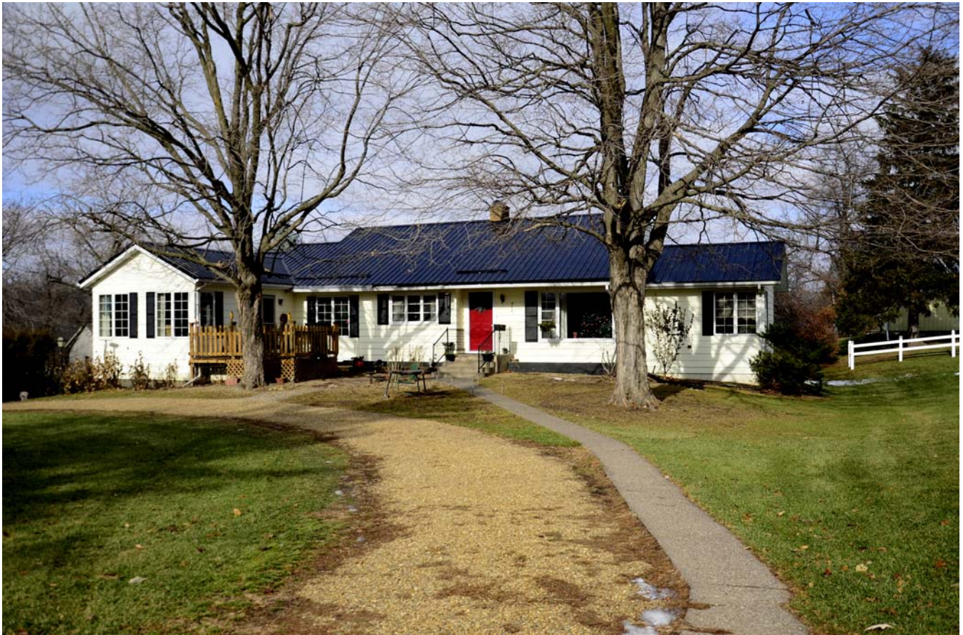
Photograph 92-00800-001 - House, looking northwest (December 2014)
