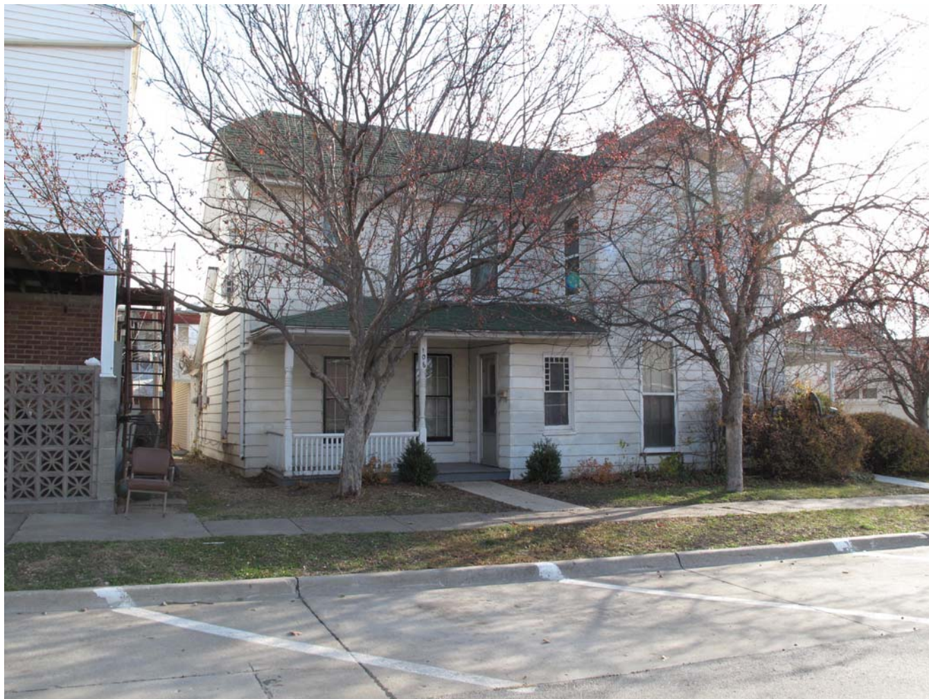
Photograph 92-00496-002 - West elevation, looking southeast (McCarley, November 15, 2011)
