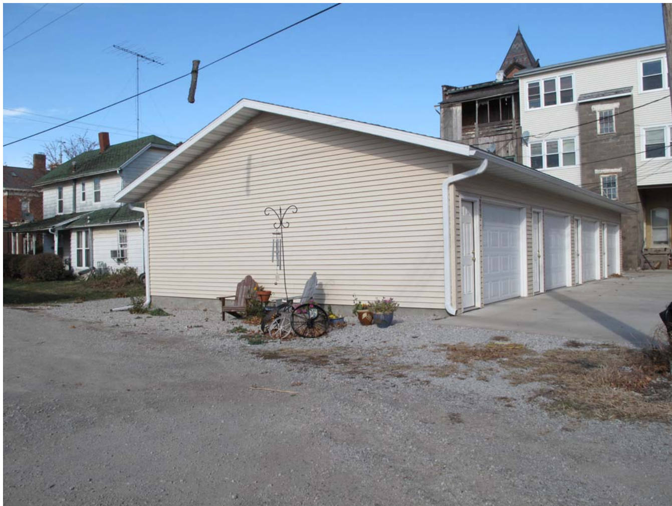
Photograph 92-00496-004 - Garage, looking northwest (McCarley, November 15, 2011)
