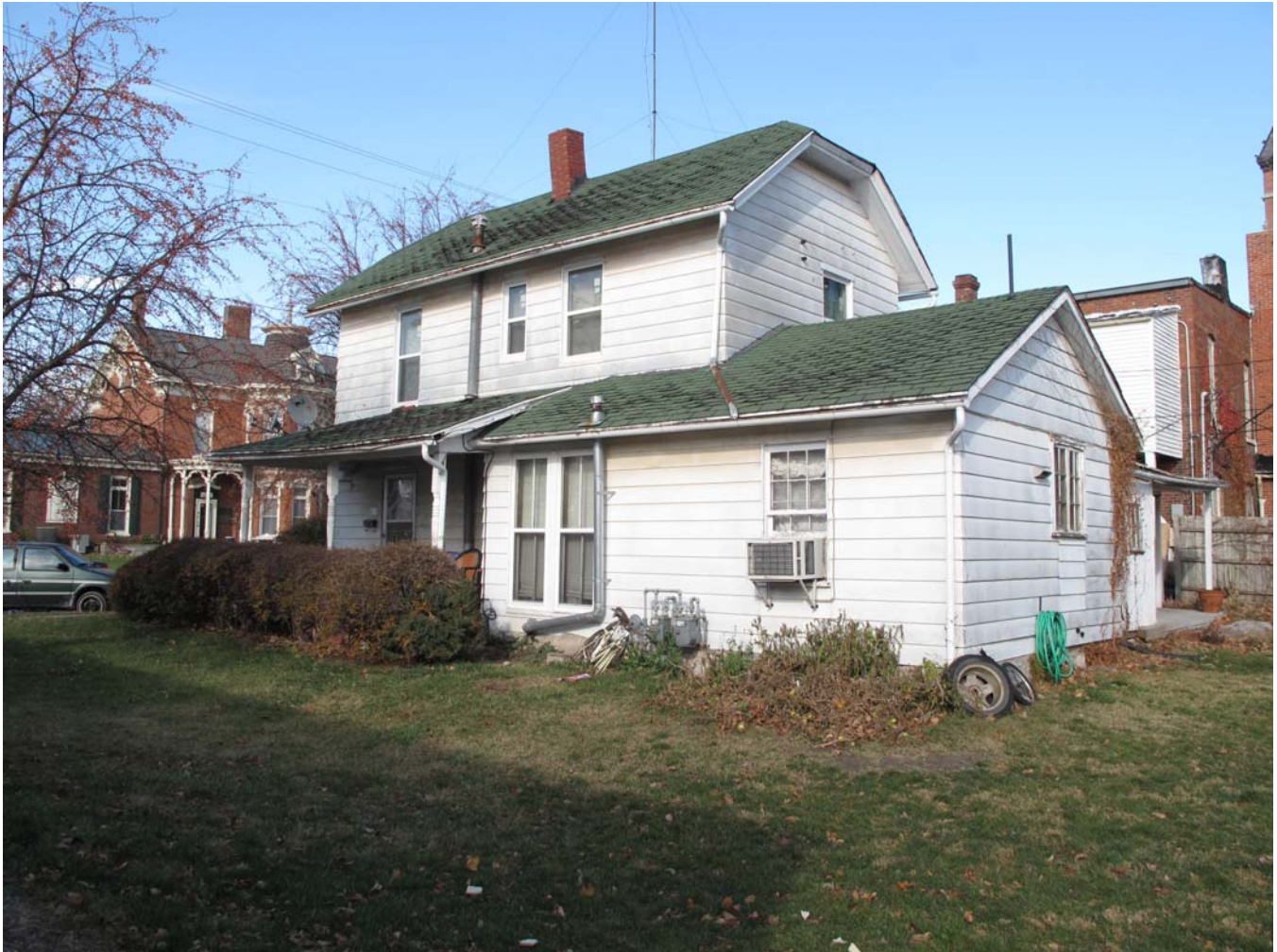
Photograph 92-00496-003 - South and east elevations, looking northwest (McCarley, November 15, 2011)
