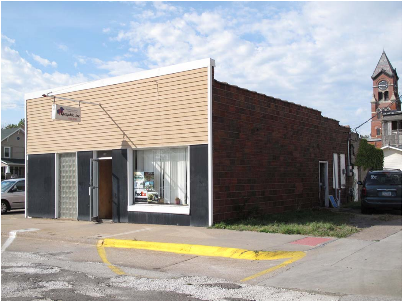
Photograph 92-00613-002 - South and east elevations, looking northwest (McCarley, September 20, 2011)
