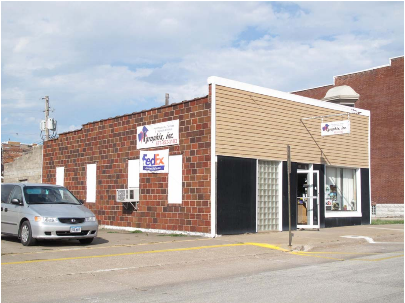
Photograph 92-00613-001 - West and south elevations, looking northeast (McCarley, September 20, 2011)
