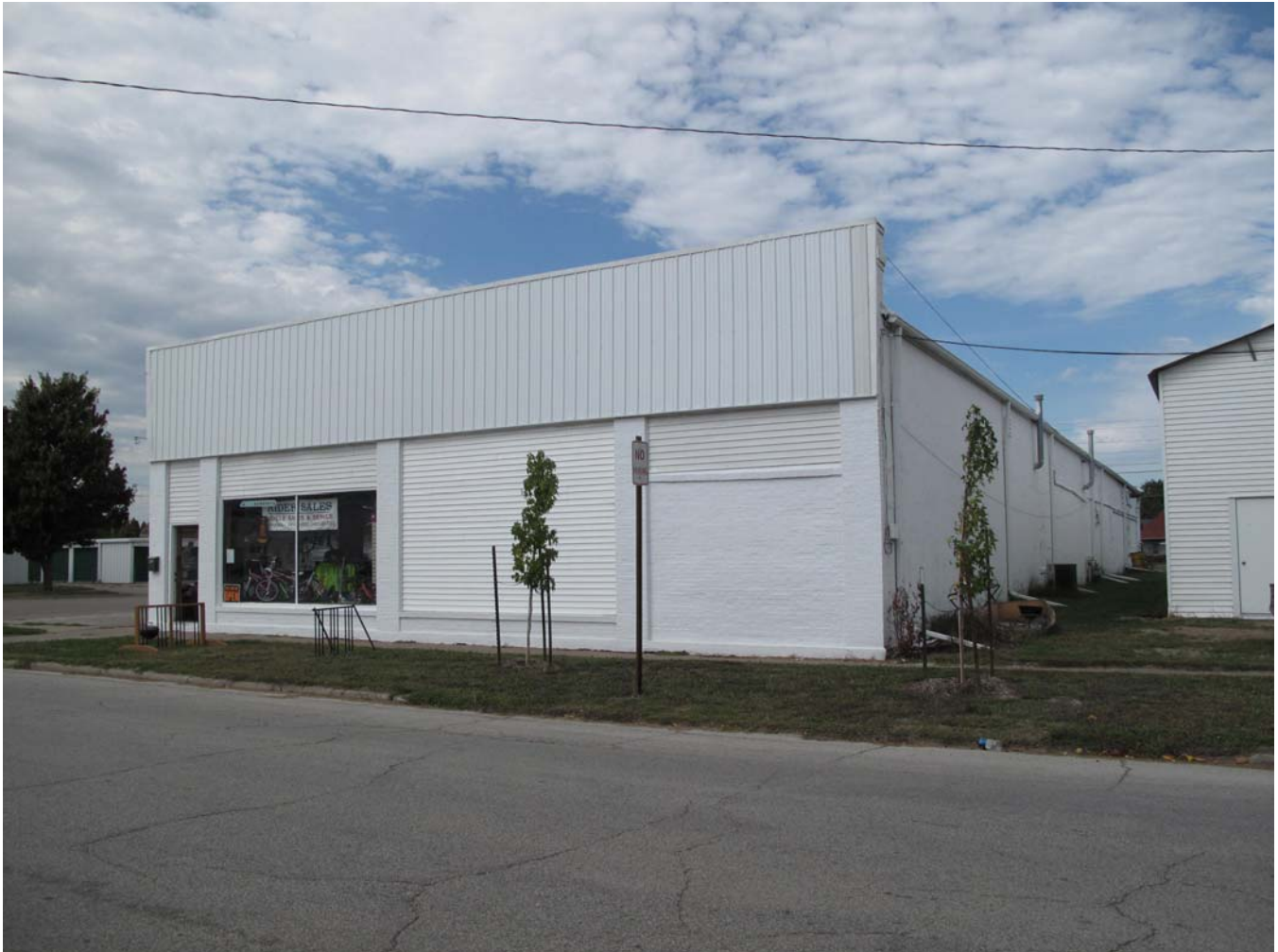
Photograph 92-00587-003 - South and east elevations, looking northwest (McCarley, September 20, 2011)
