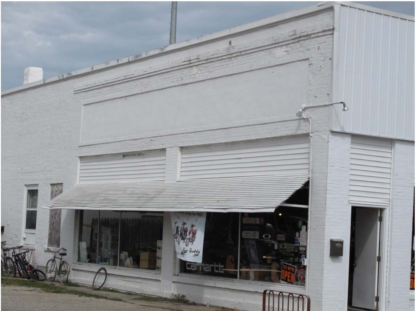
Photograph 92-00587-002 - Detail of brick on west elevation, looking northeast (McCarley, September 20, 2011)
