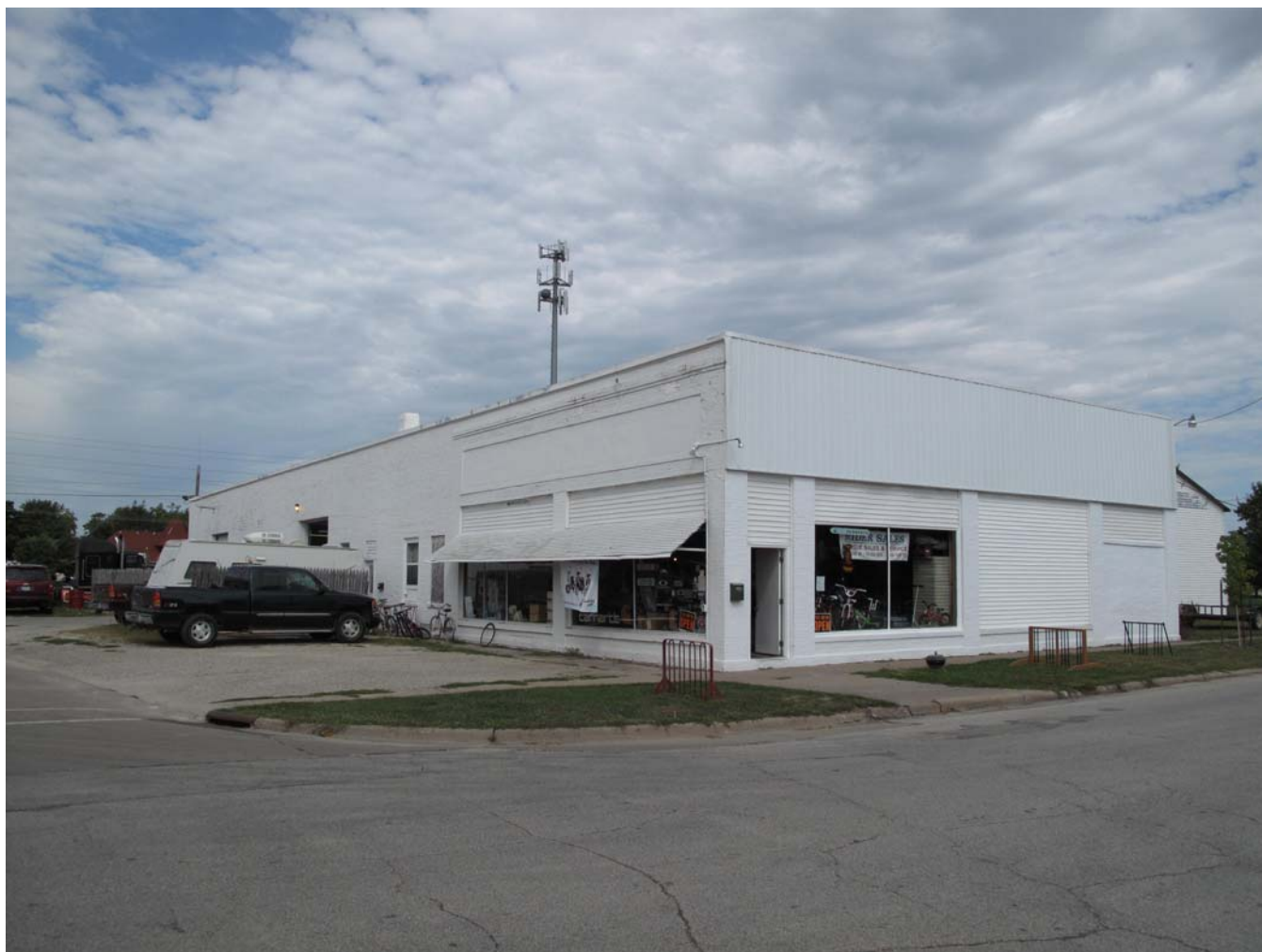
Photograph 92-00587-001 - West and south elevations, looking northeast (McCarley, September 20, 2011)
