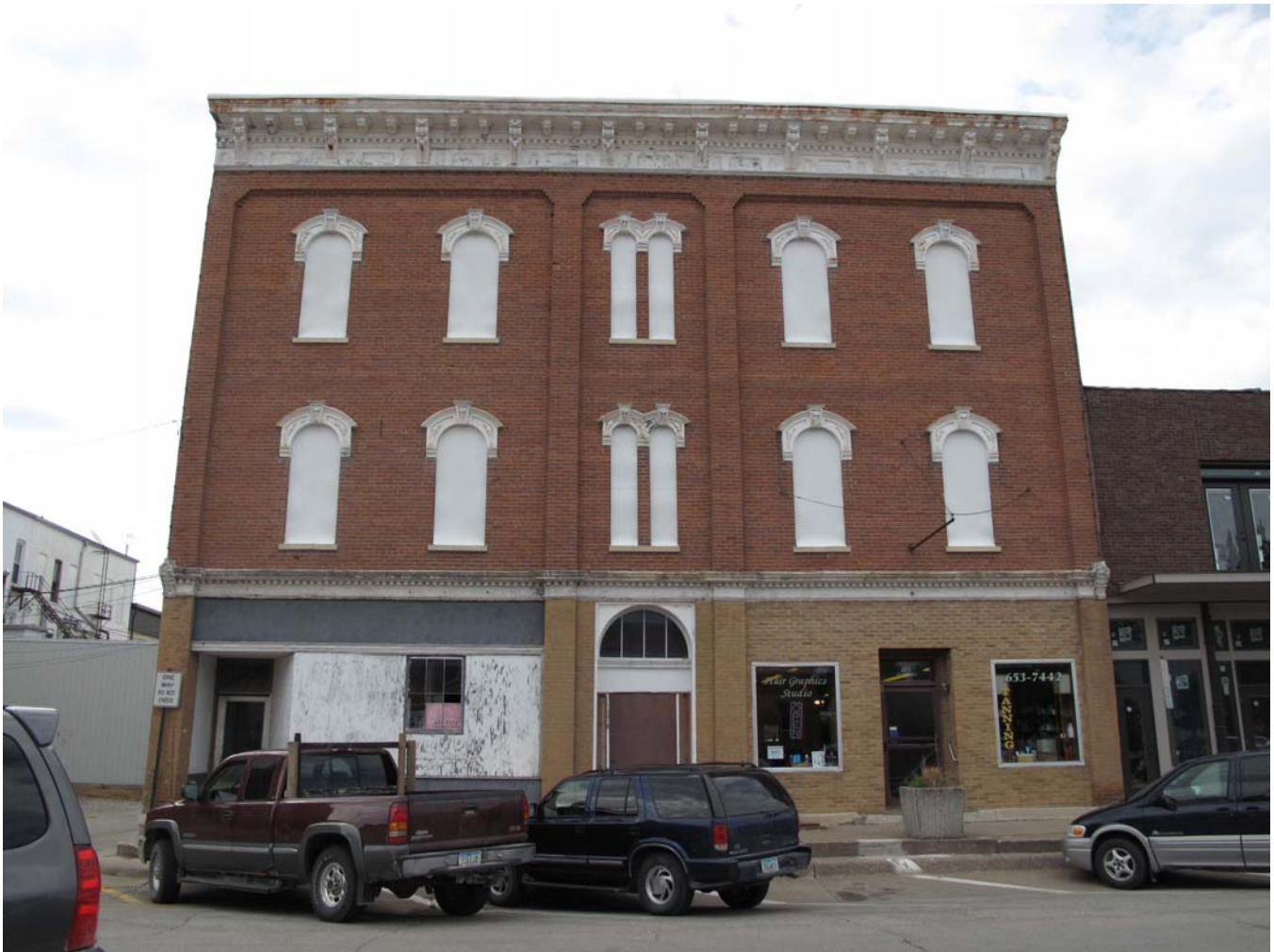
Photograph 92-00502-002 - East elevation, looking west (McCarley, September 20, 2011)
