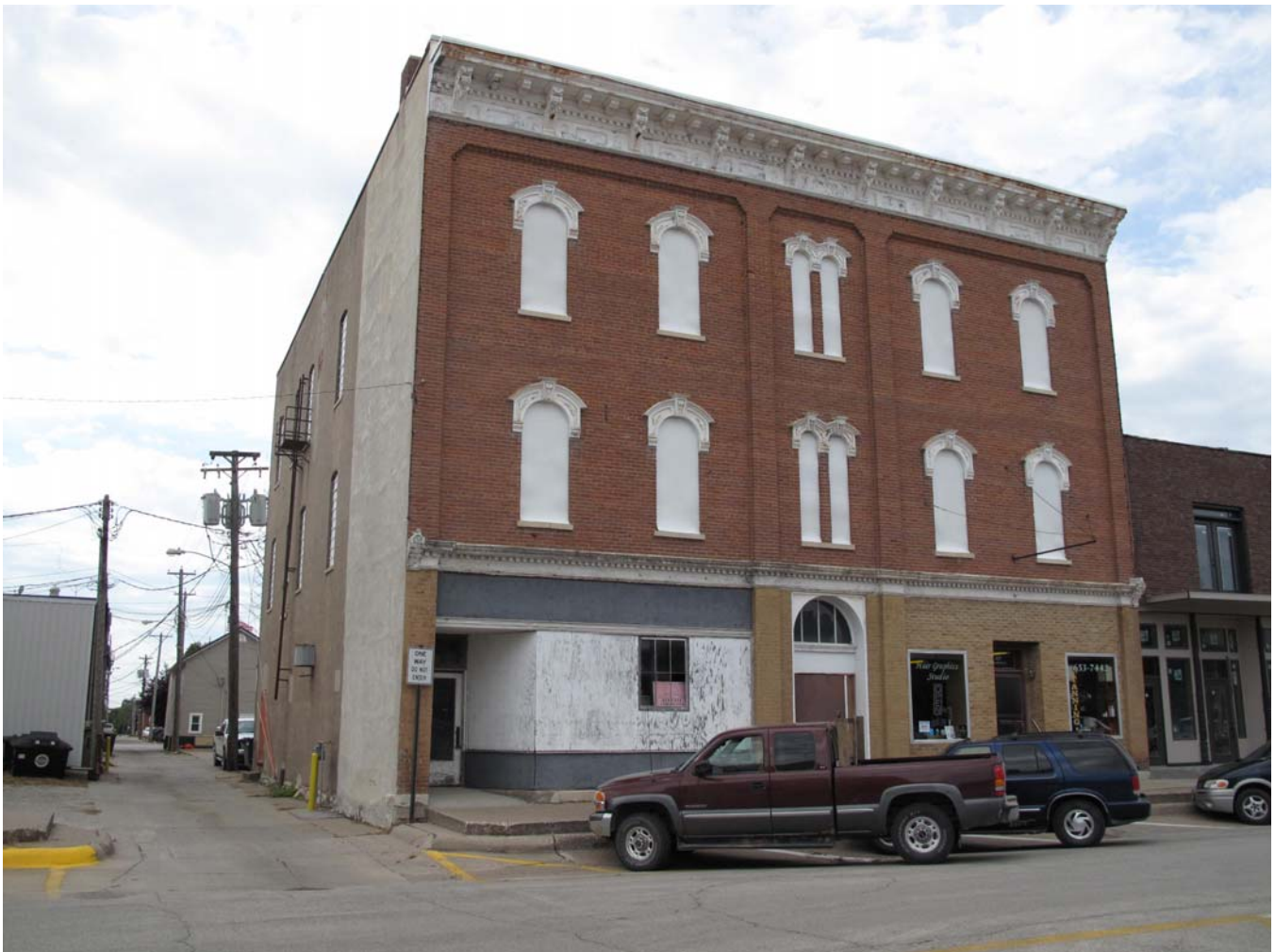
Photograph 92-00502-001 - East elevation, looking northwest (McCarley, September 20, 2011)
