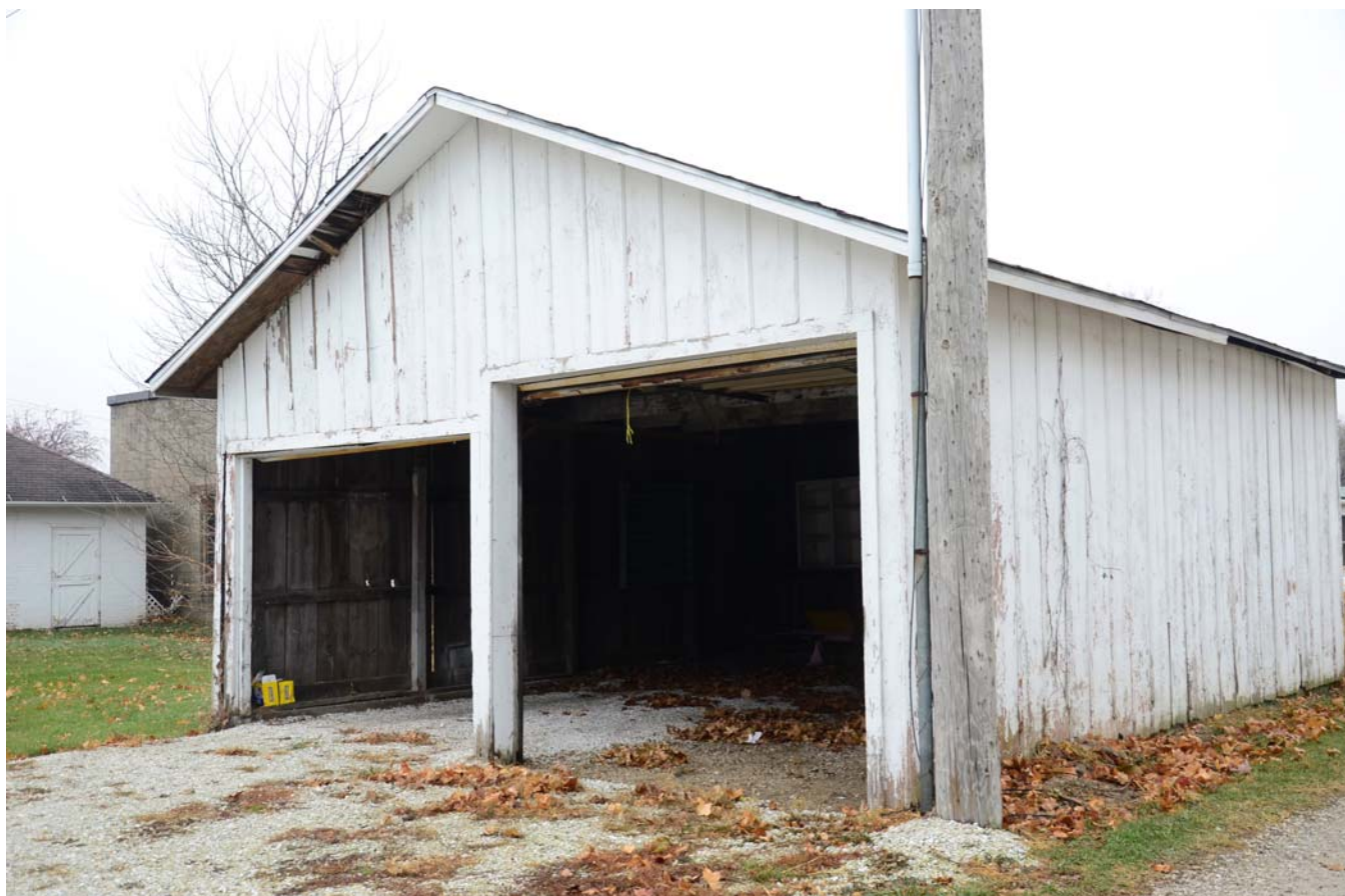
Photograph 92-00428-004 - Garage, looking southwest (December 2014)
