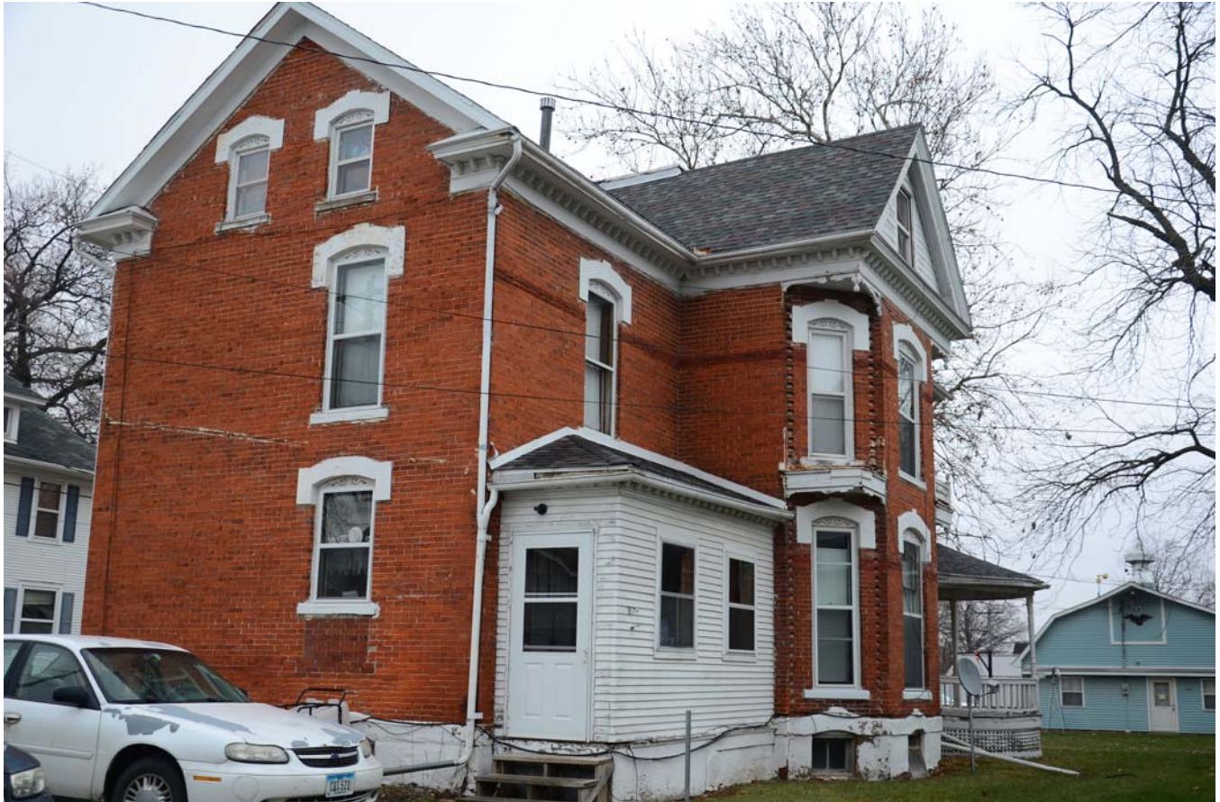
Photograph 92-00428-003 - House, looking northeast (December 2014)
