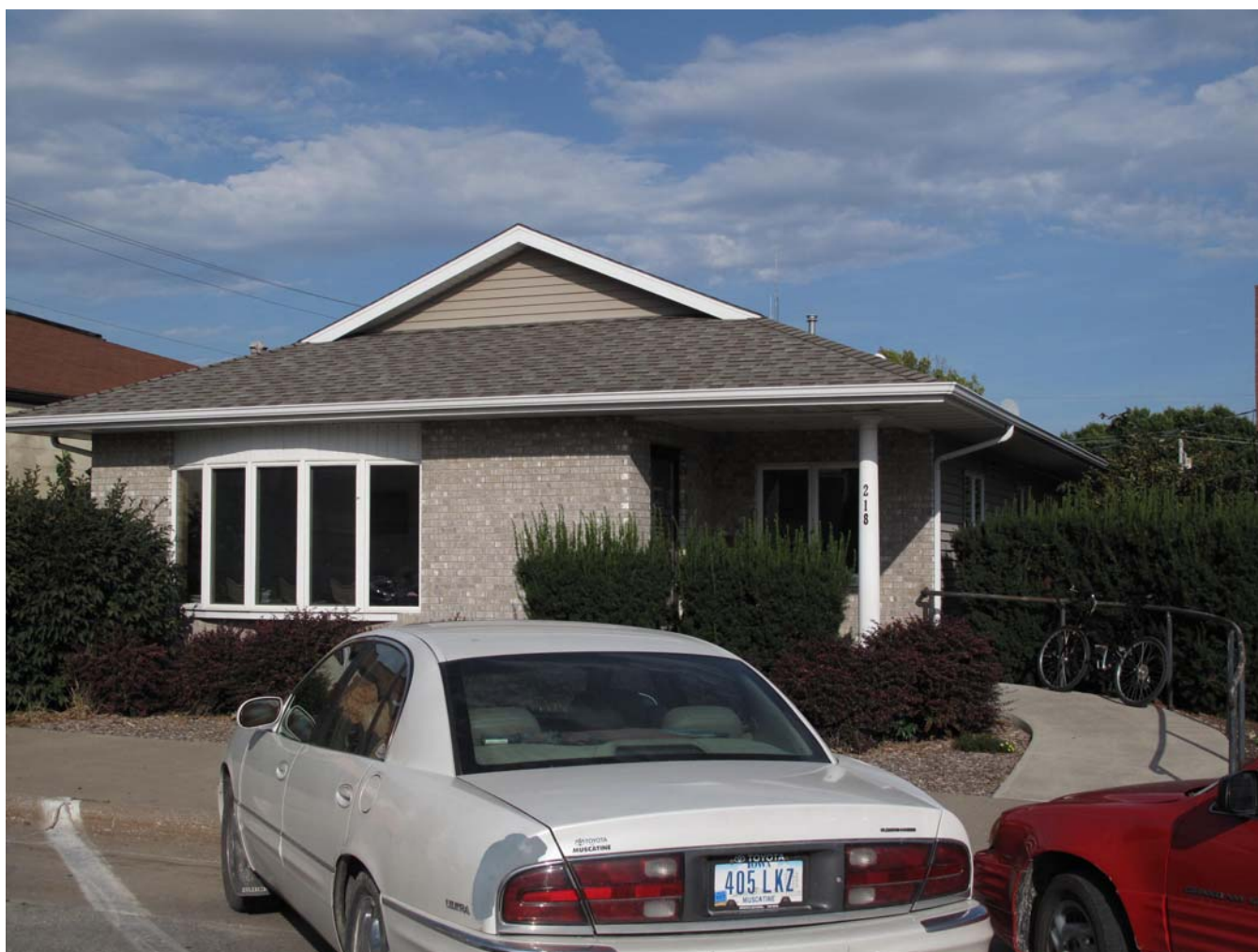
Photograph 92-00524-001 - West and south elevations, looking northeast (McCarley, September 20, 2011)
