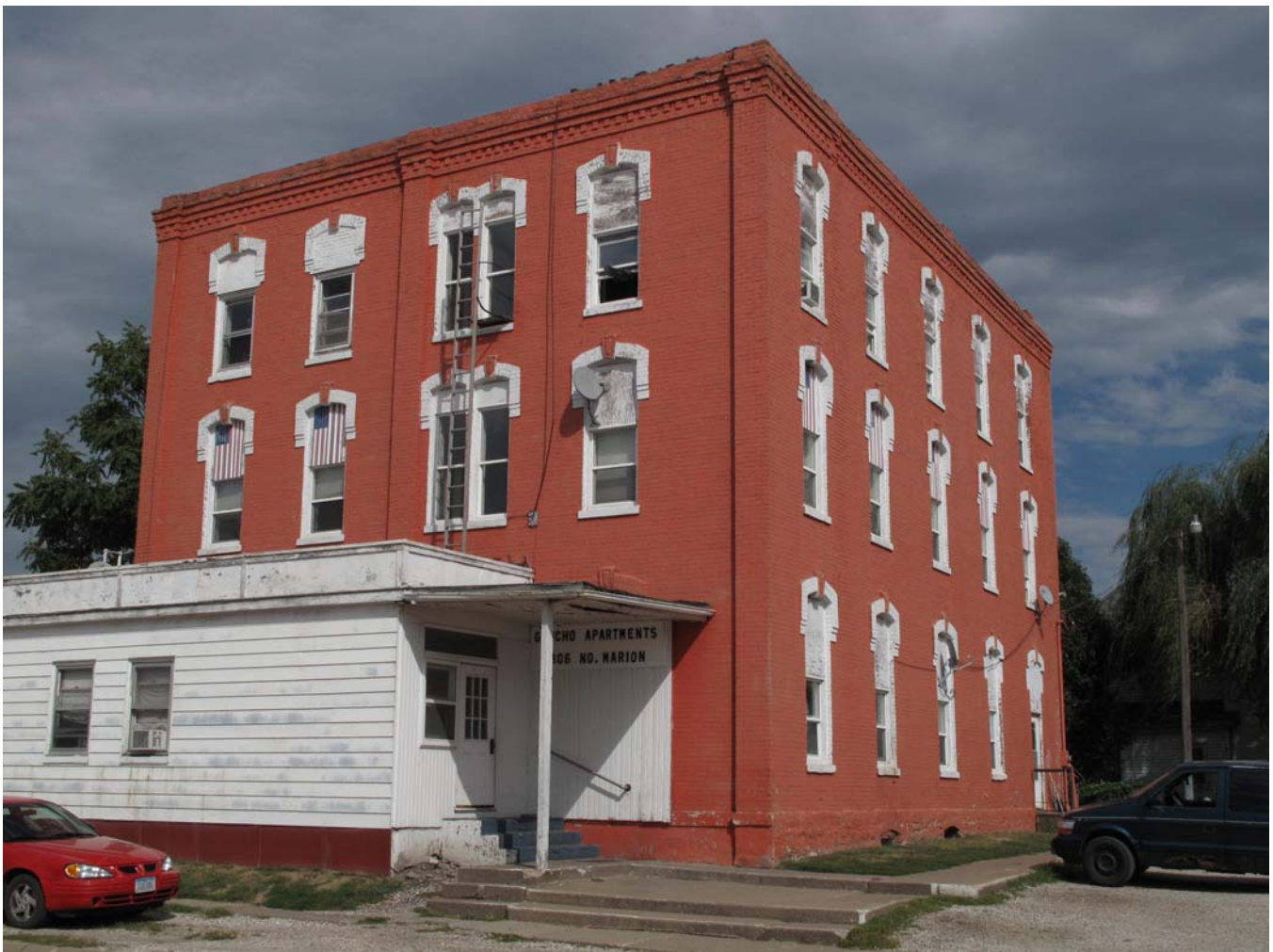
Photograph 92-00664-001 - West and south elevations, looking northeast (McCarley, September 20, 2011)
