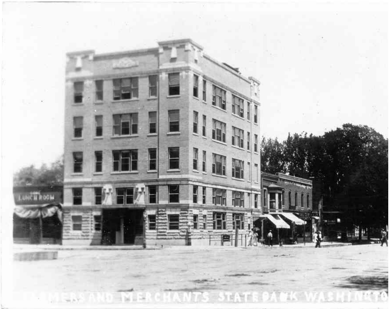
Building around 1915 (Patterson collection).
