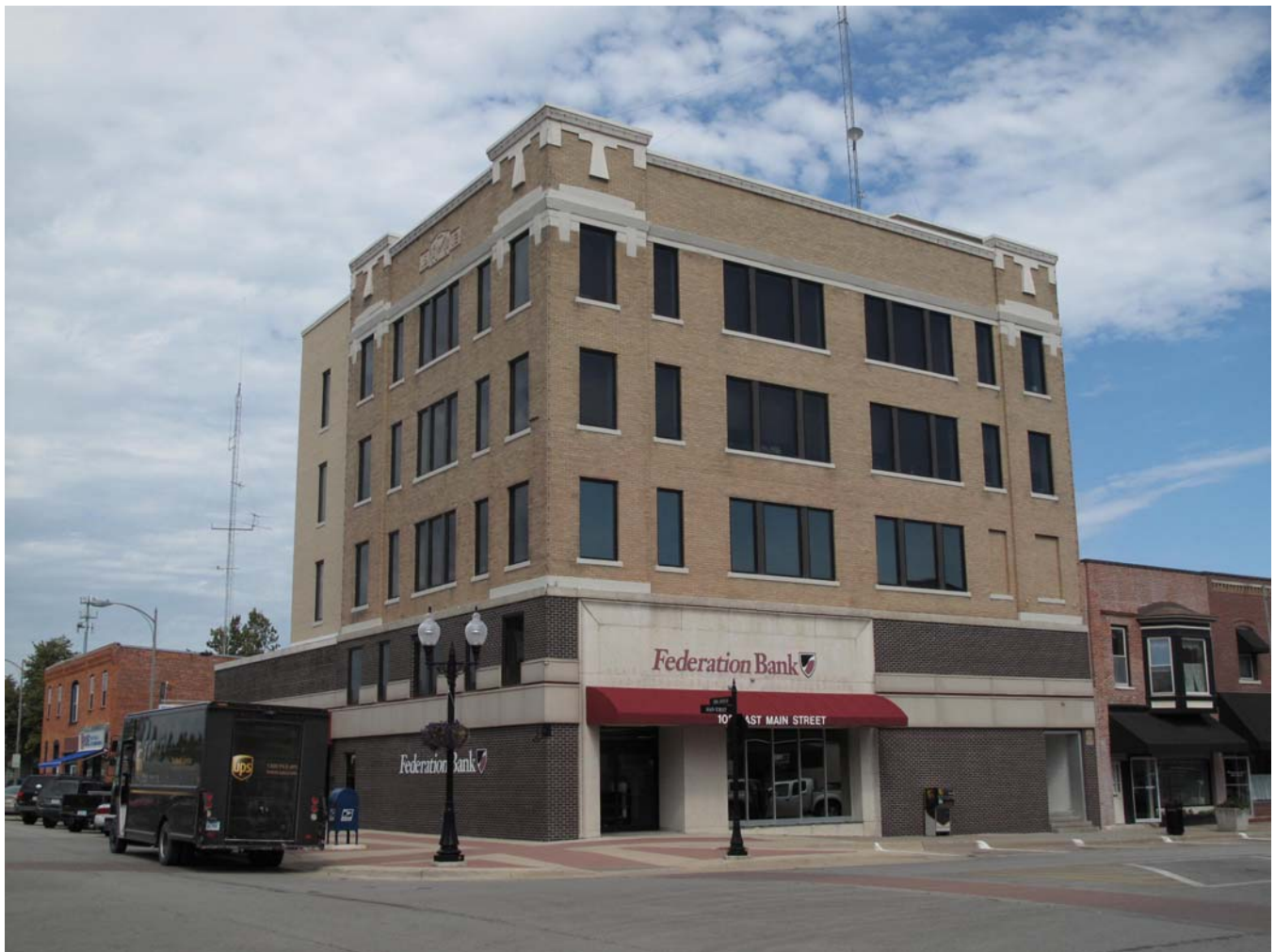
Photograph 92-00548-001 - West and south elevations, looking northeast (McCarley, September 20, 2011).
