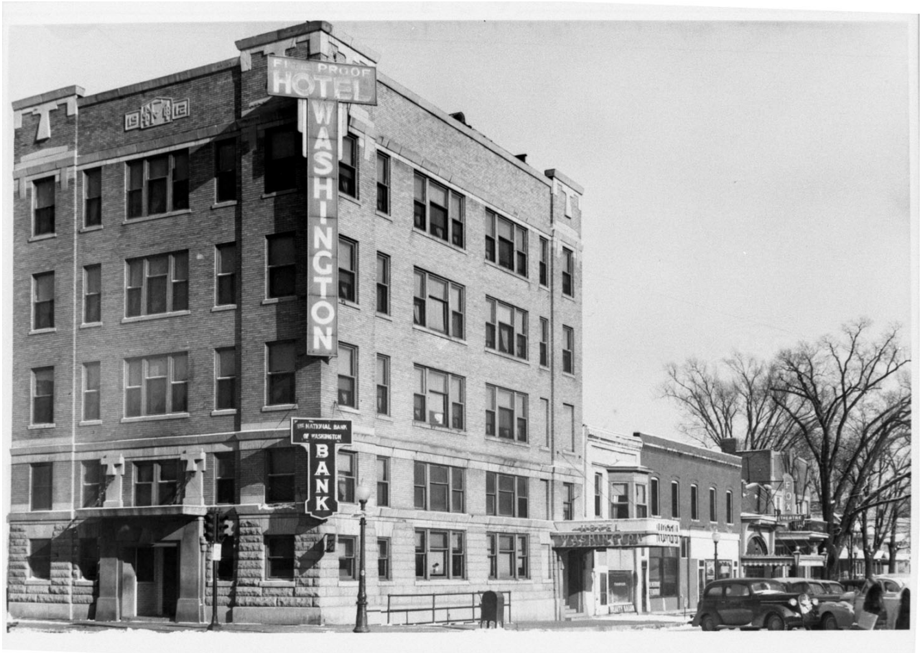
Photograph of building in 1930s (Patterson collection).
