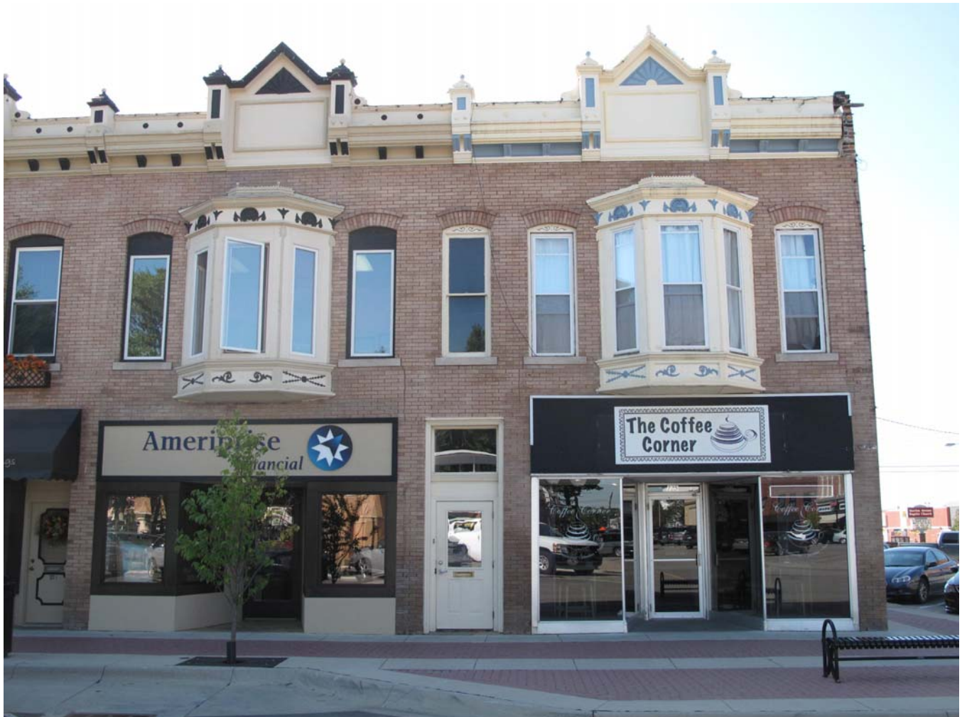
Photograph 92-00607-002 - North elevation of 123-125 W. Washington, looking south (McCarley, September 20, 2011)
