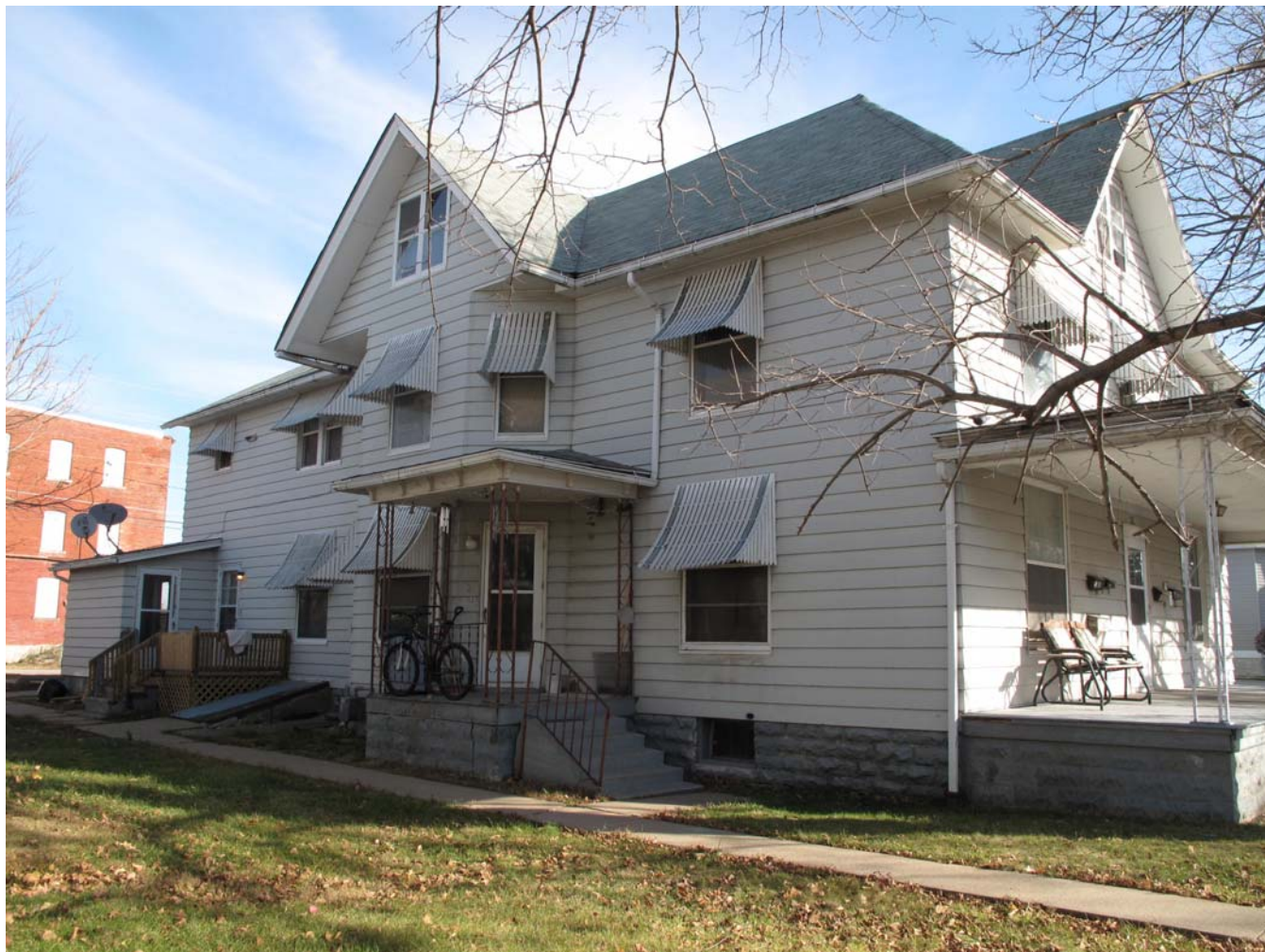
Photograph 92-00577-002 - West and south elevations, looking northeast (McCarley, November 15, 2011)
