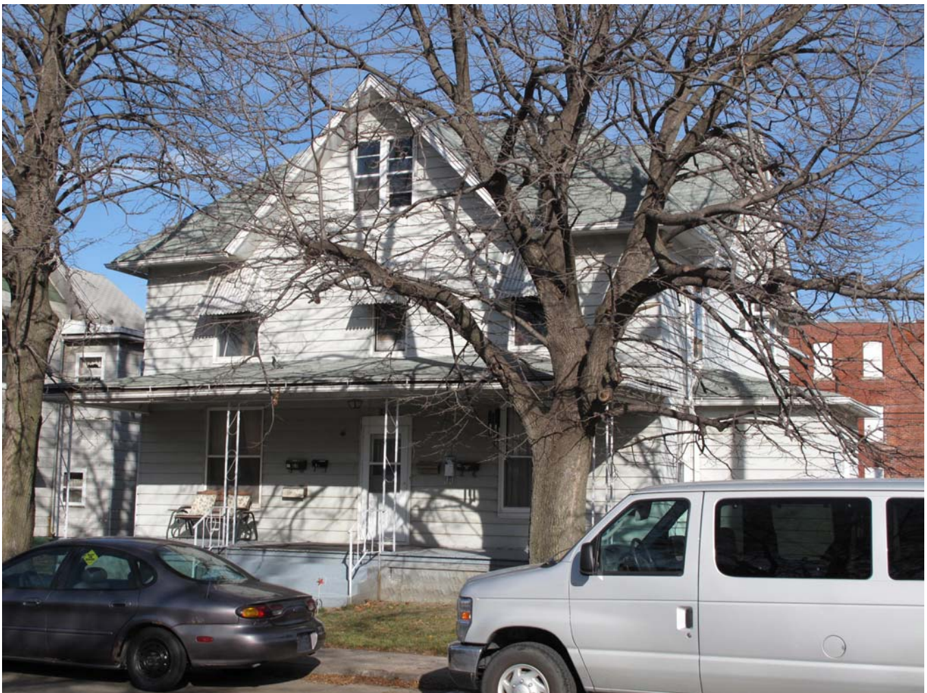
Photograph 92-00577-001 - South and east elevations, looking northwest (McCarley, November 15, 2011)
