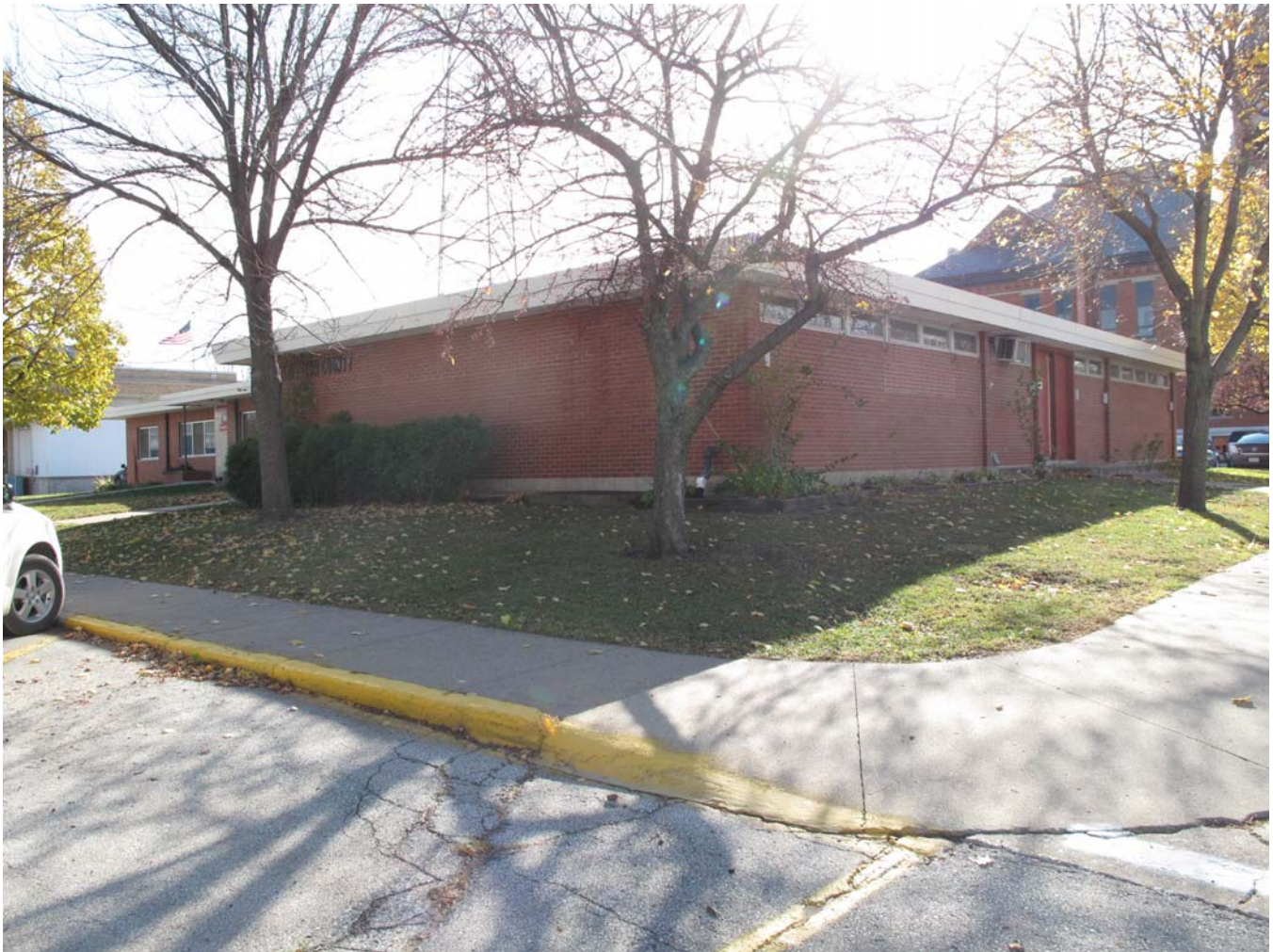
Photograph 92-00585-005 - North and west elevations, looking southeast (McCarley, November 15, 2011).
