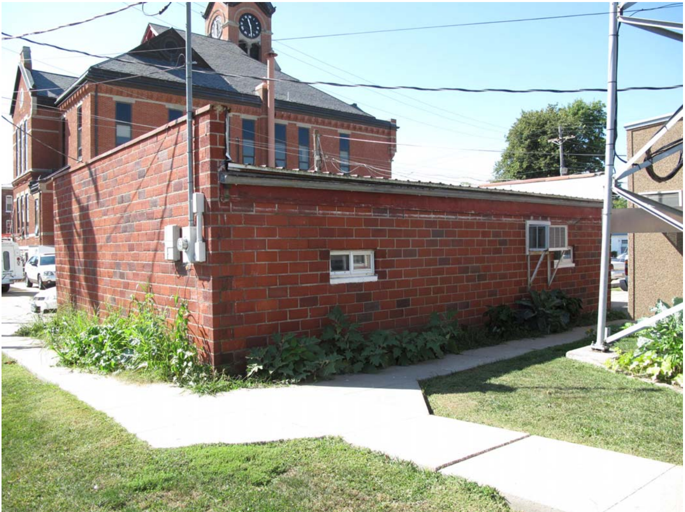
Photograph 92-00585-009 - Tile block garage, looking southwest (McCarley, November 15, 2011).
