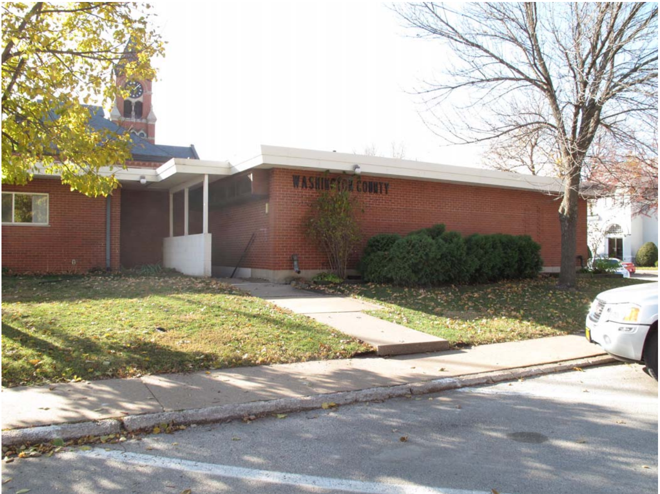
Photograph 92-00585-004 - East and north elevations of west/jail section, looking southwest (McCarley, November 15, 2011).
