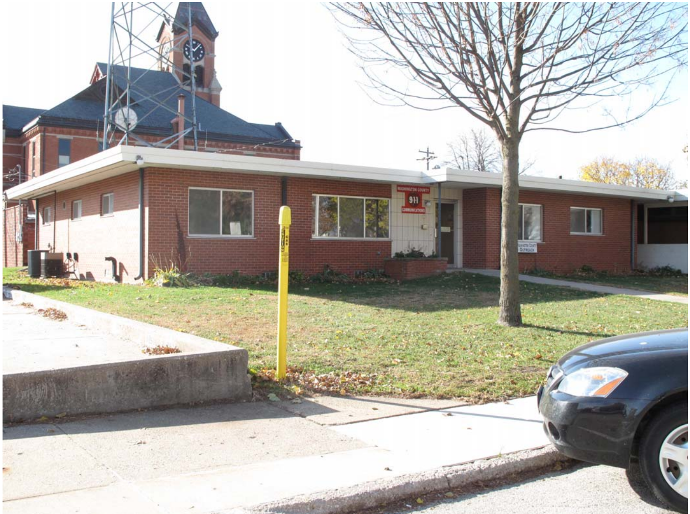
Photograph 92-00585-003 - East and north elevations of east/office section, looking southwest (McCarley, November 15, 2011).
