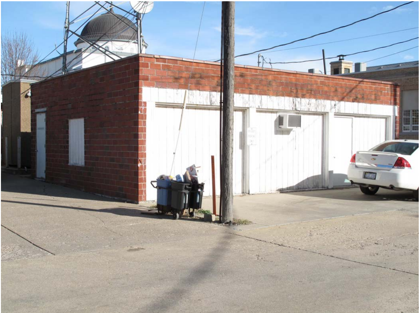
Photograph 92-00585-008 - Tile block garage, looking northeast (McCarley, November 15, 2011).
