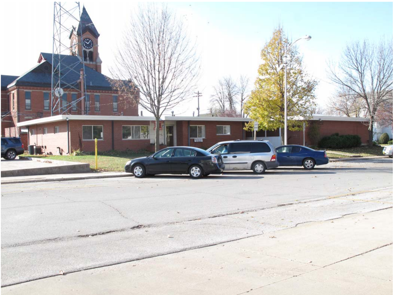
Photograph 92-00585-001 - East and north elevations, looking southwest (McCarley, November 15, 2011).
