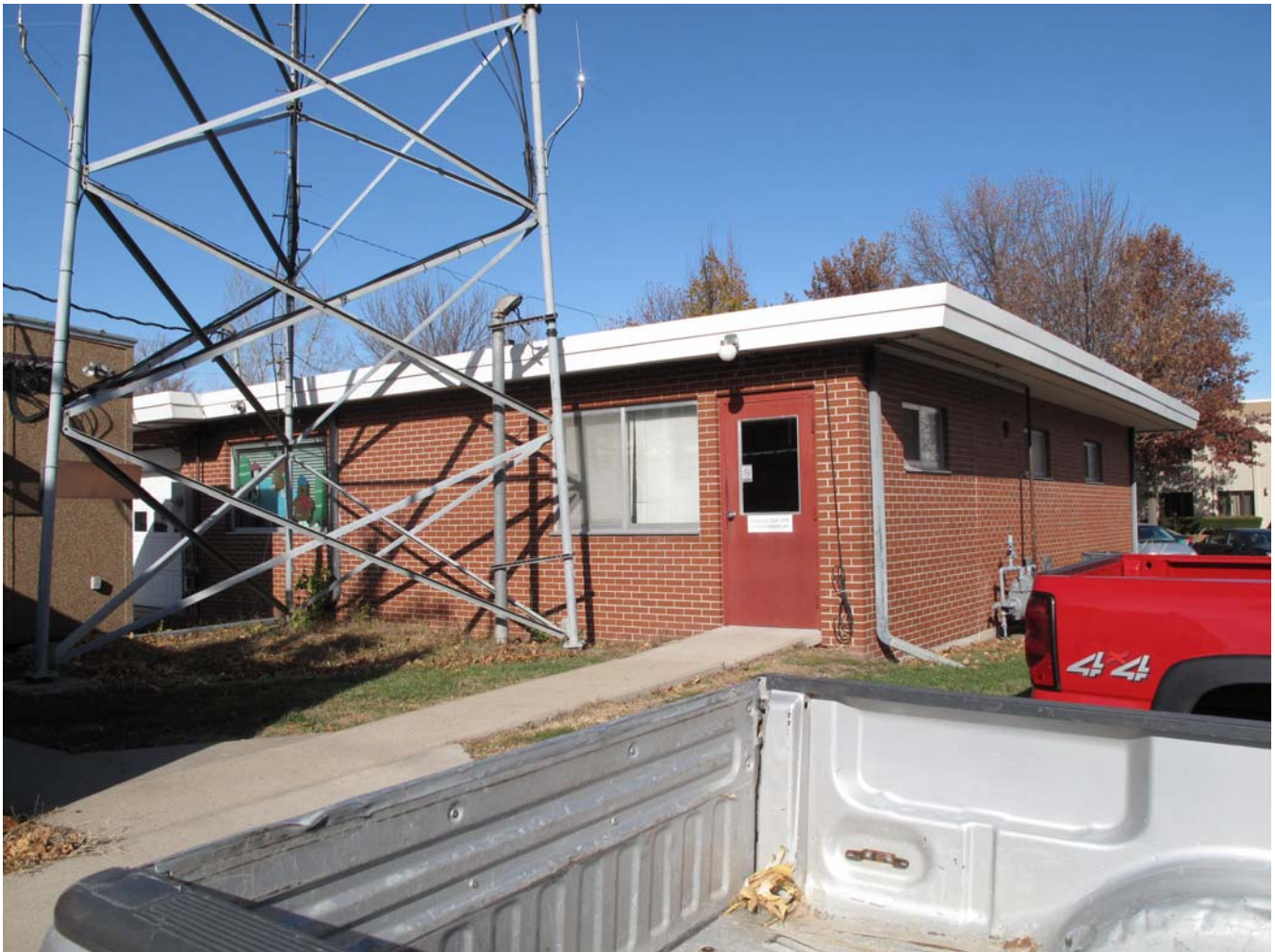
Photograph 92-00585-007 - South elevation of east section, looking northwest (McCarley, November 15, 2011).
