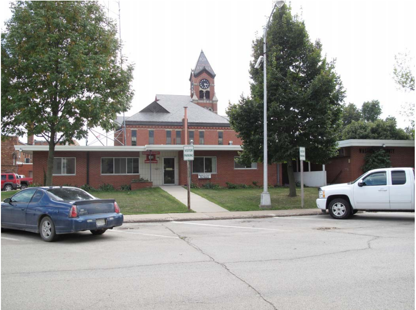
Photograph 92-00585-002 - North elevation, looking south (McCarley, November 15, 2011).
