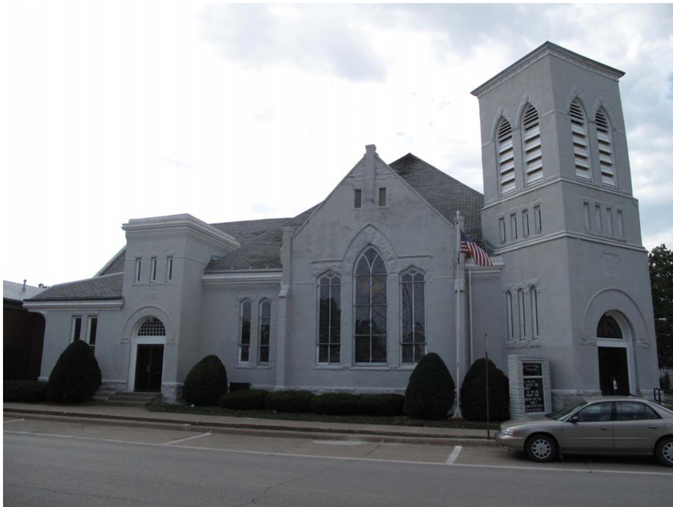
Photograph 92-00347-002 - East elevation, looking west (McCarley, September 20, 2011).
