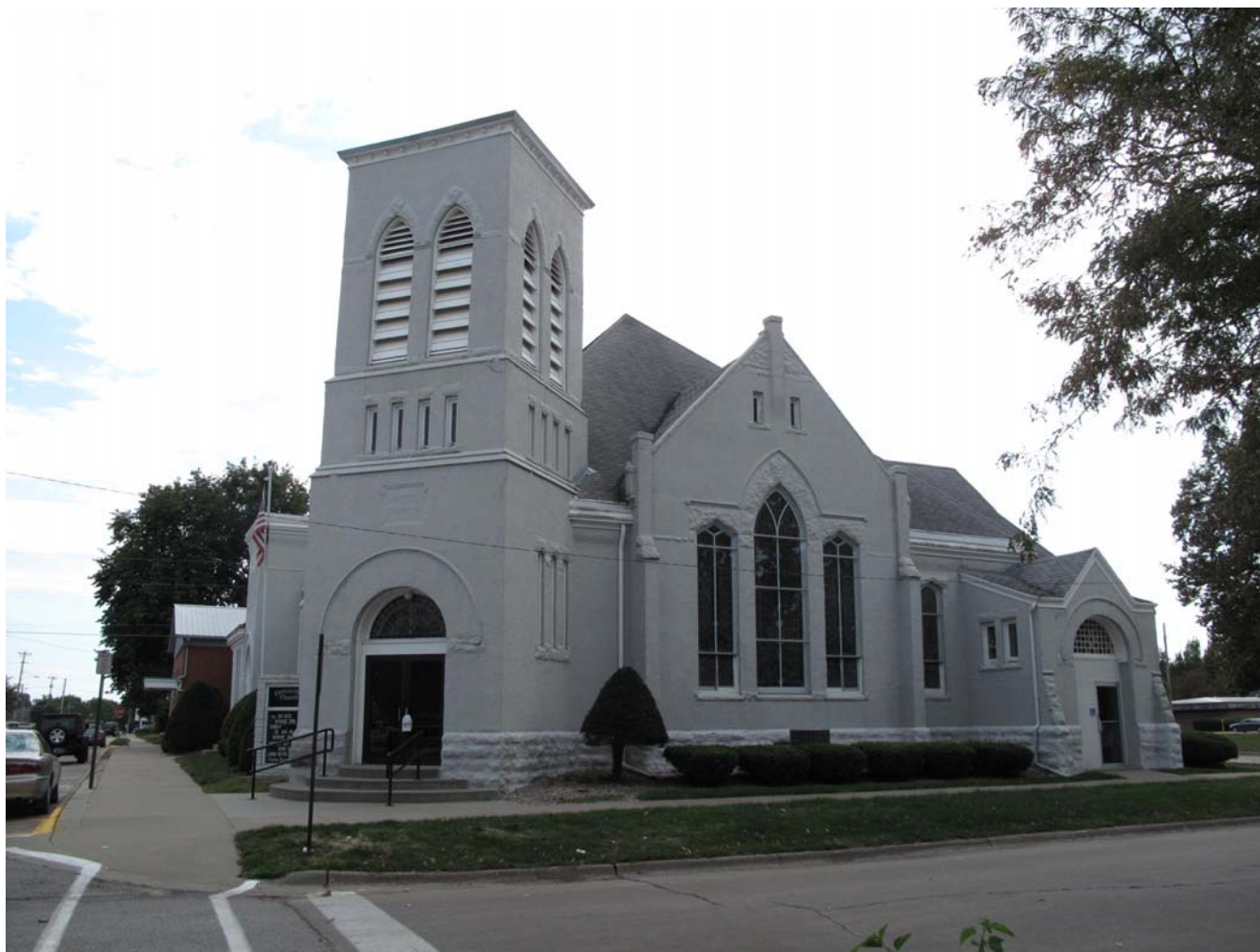
Photograph 92-00347-001 - North elevation, looking south-southwest (McCarley, September 20, 2011).
