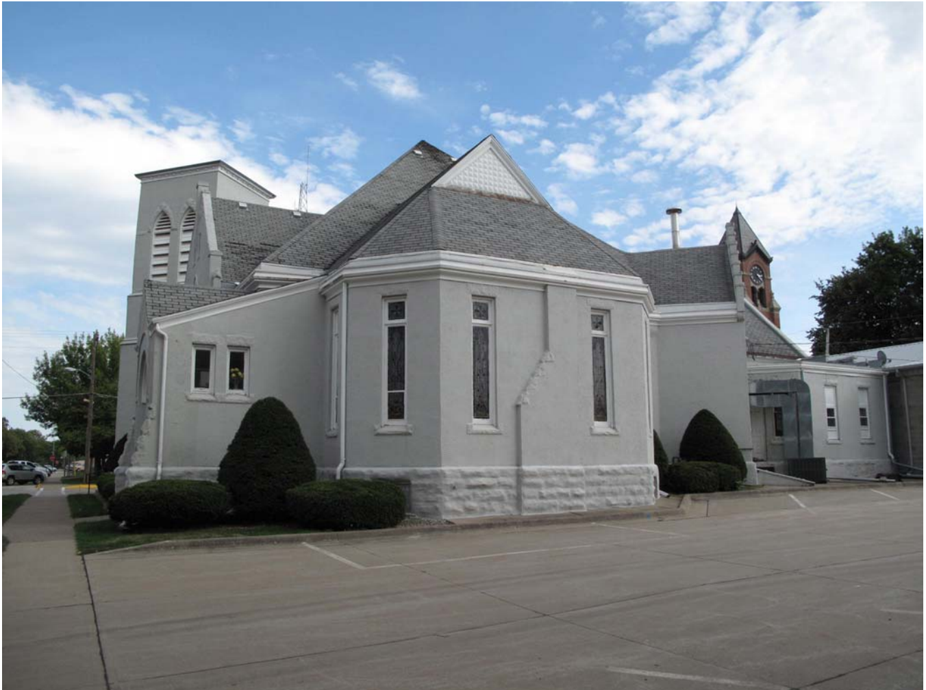
Photograph 92-00347-004 - West elevation, looking east (McCarley, September 20, 2011).
