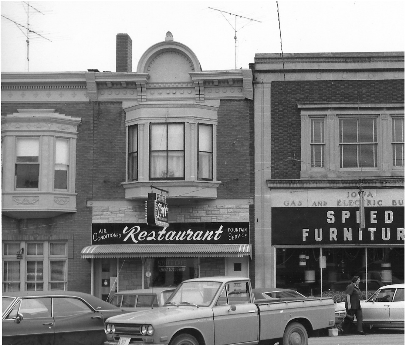
Building in 1971 (Wagner 1971)
