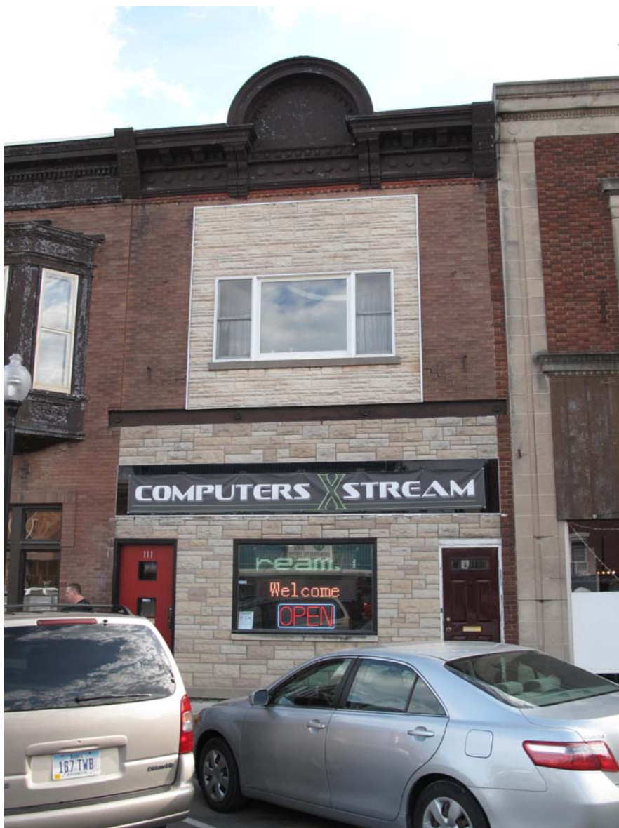
Photograph 92-00594-001 - North elevation, looking south (McCarley, September 20, 2011)
