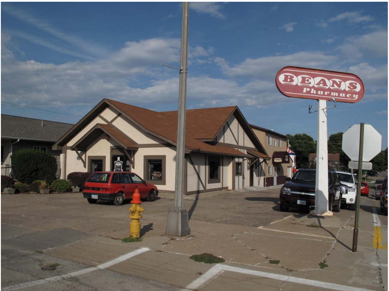
Photograph 92-00528-001 - West and south elevations, looking northeast (McCarley, September 20, 2011)
