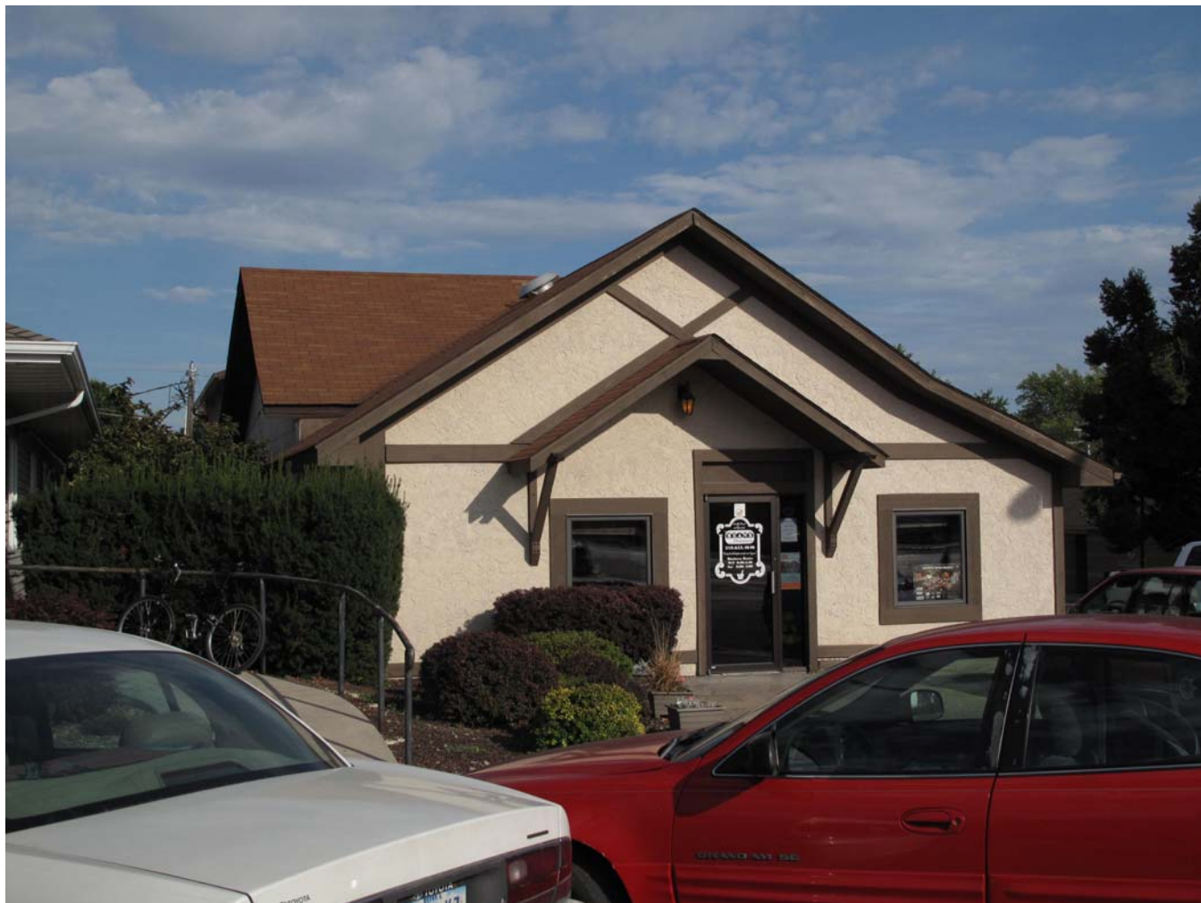
Photograph 92-00528-003 - West elevation, looking east (McCarley, September 20, 2011)
