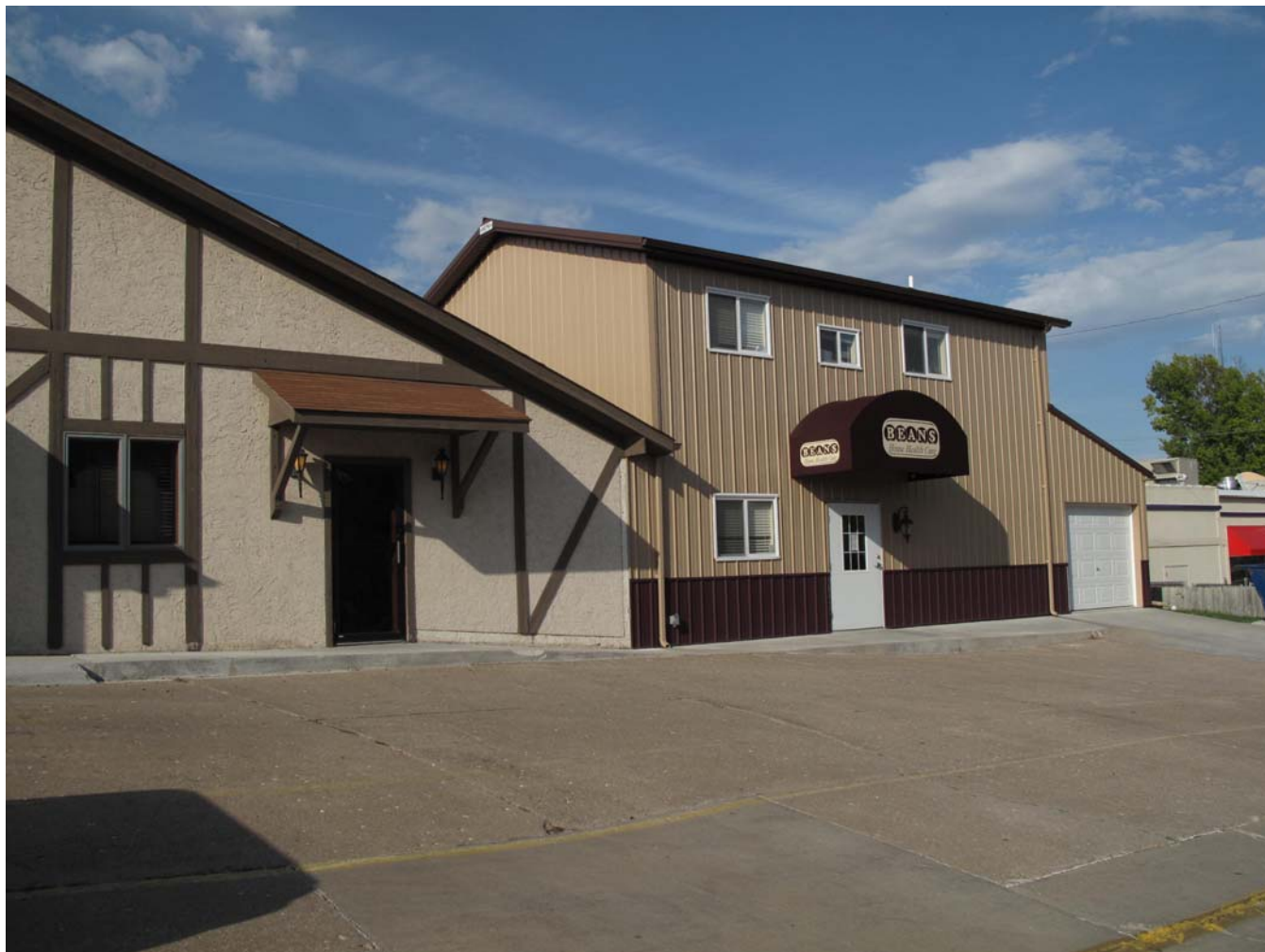
Photograph 92-00528-004 - South side of east addition, looking northeast (McCarley, September 20, 2011)
