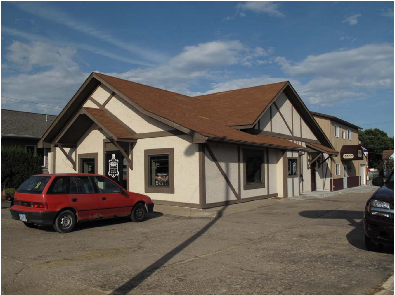
Photograph 92-00528-002 - West and south elevations, looking northeast (McCarley, September 20, 2011)
