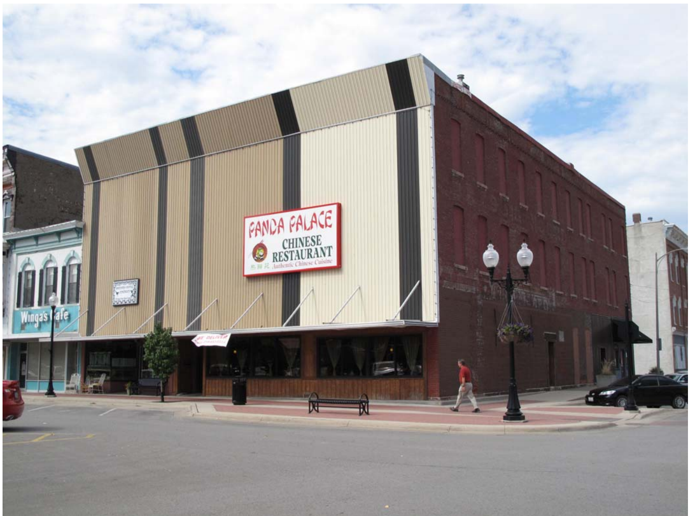
Photograph 92-00538-001 - South and east elevations, looking northwest (McCarley, September 20, 2011).
