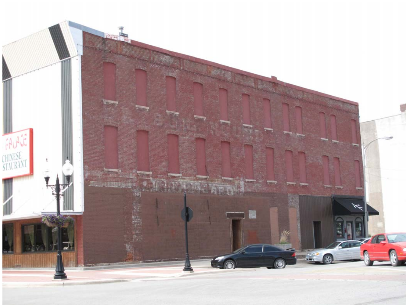
Photograph 92-00538-002 - East elevation, looking northwest (McCarley, September 20, 2011).
