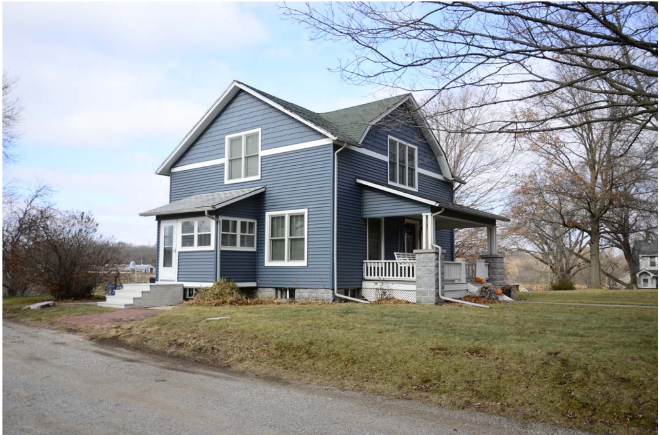
Photograph 92-00803-002 - House, looking northwest (December 2014)
