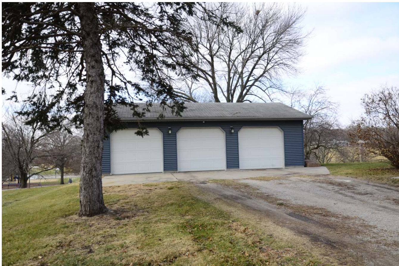
Photograph 92-00803-004 - Garage, looking west (December 2014)
