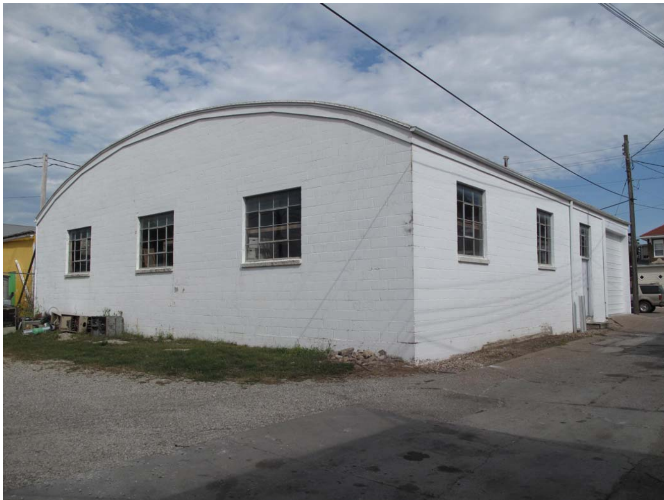
92-00662-002 - West and south elevations, looking northeast (McCarley, September 20, 2011)
