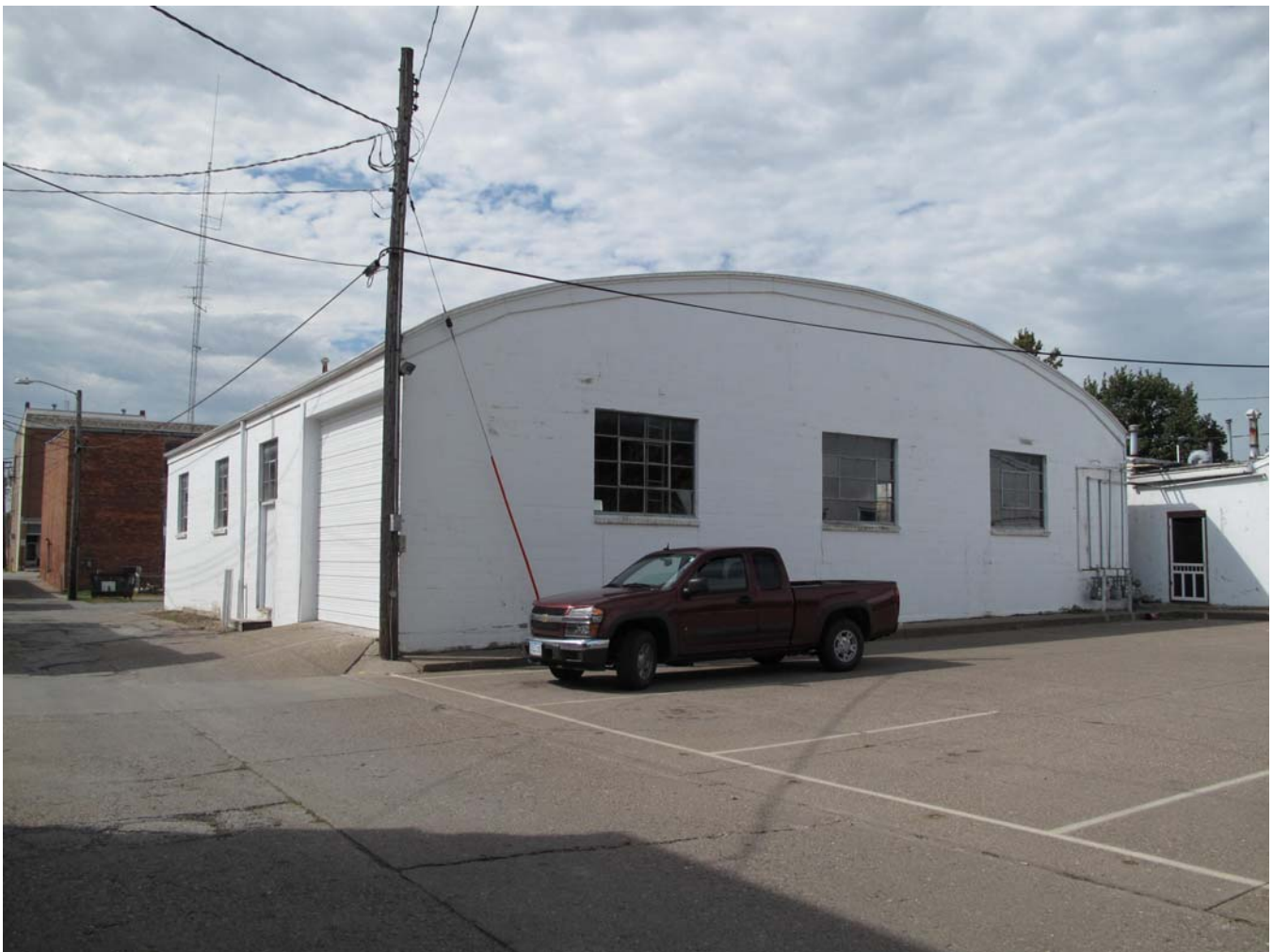
92-00662-001 - South and east elevations, looking northwest (McCarley, September 20, 2011)
