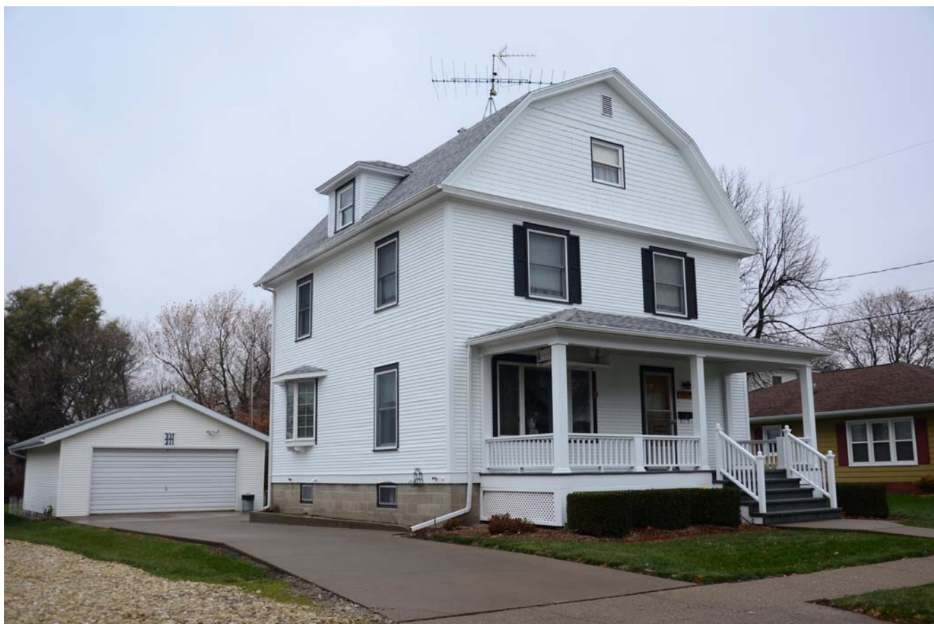
Photograph 92-00738-001 - House, looking northwest (December 2014)
