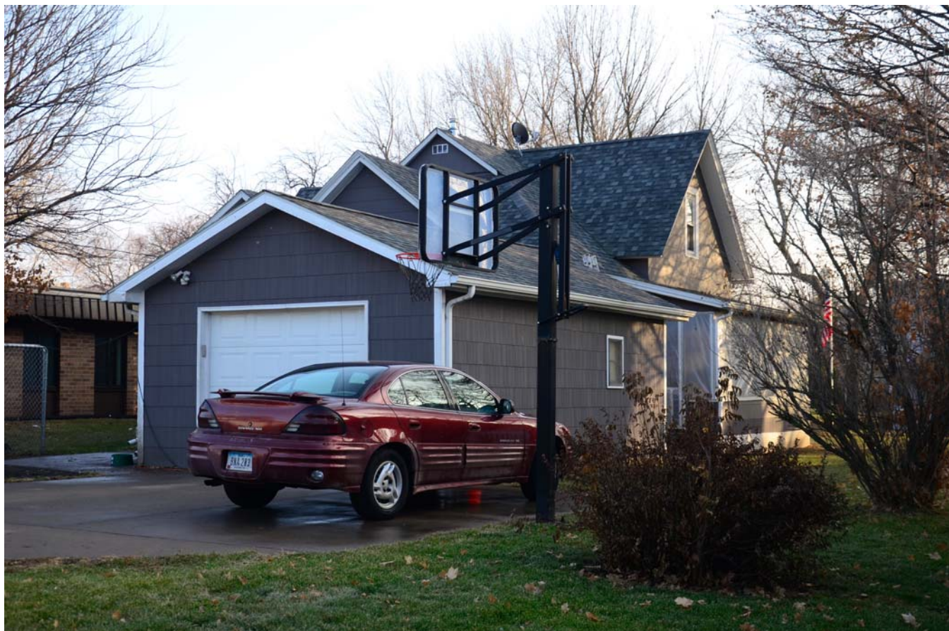
Photograph 92-00414-004 - House, looking southeast (December 2014)
