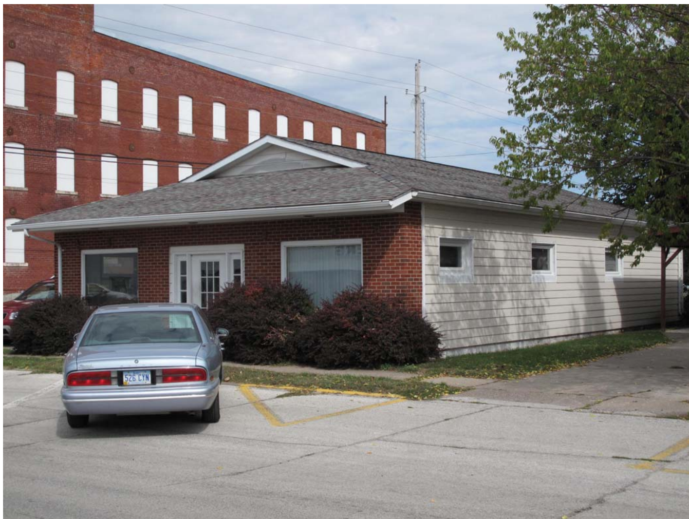
Photograph 92-00505-001 - West and south elevations, looking northeast (McCarley, September 20, 2011)
