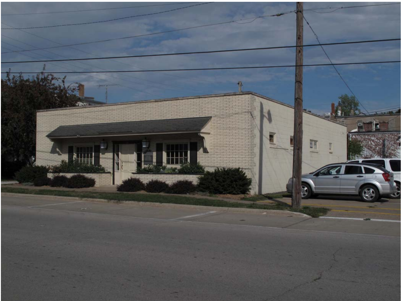
Photograph 92-00497-001 - West and south elevations, looking northeast (McCarley, September 20, 2011)
