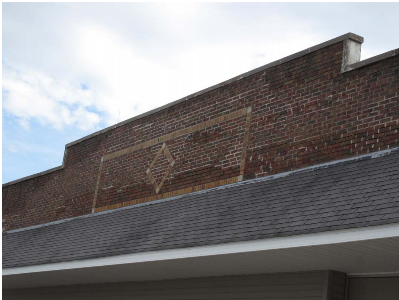
Photograph 92-00581-002 - Detail on north elevation, looking southeast (McCarley, September 20, 2011)
