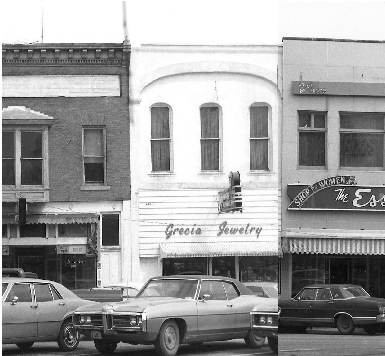
Building in 1971 (Wagner 1971)
