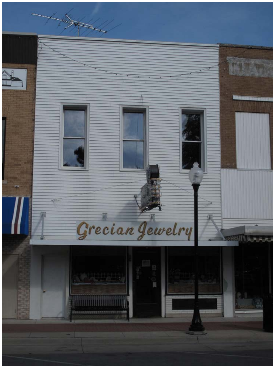
Photograph 56-00510-001 - West elevation, looking east (McCarley, September 20, 2011)
