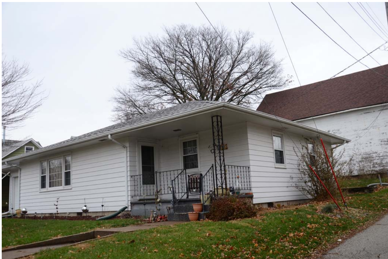
Photograph 92-00729-001 - House, looking northeast (December 2014)
