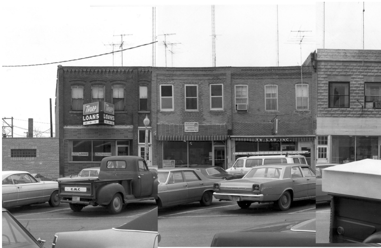
Building in 1971 (Wagner 1971)
