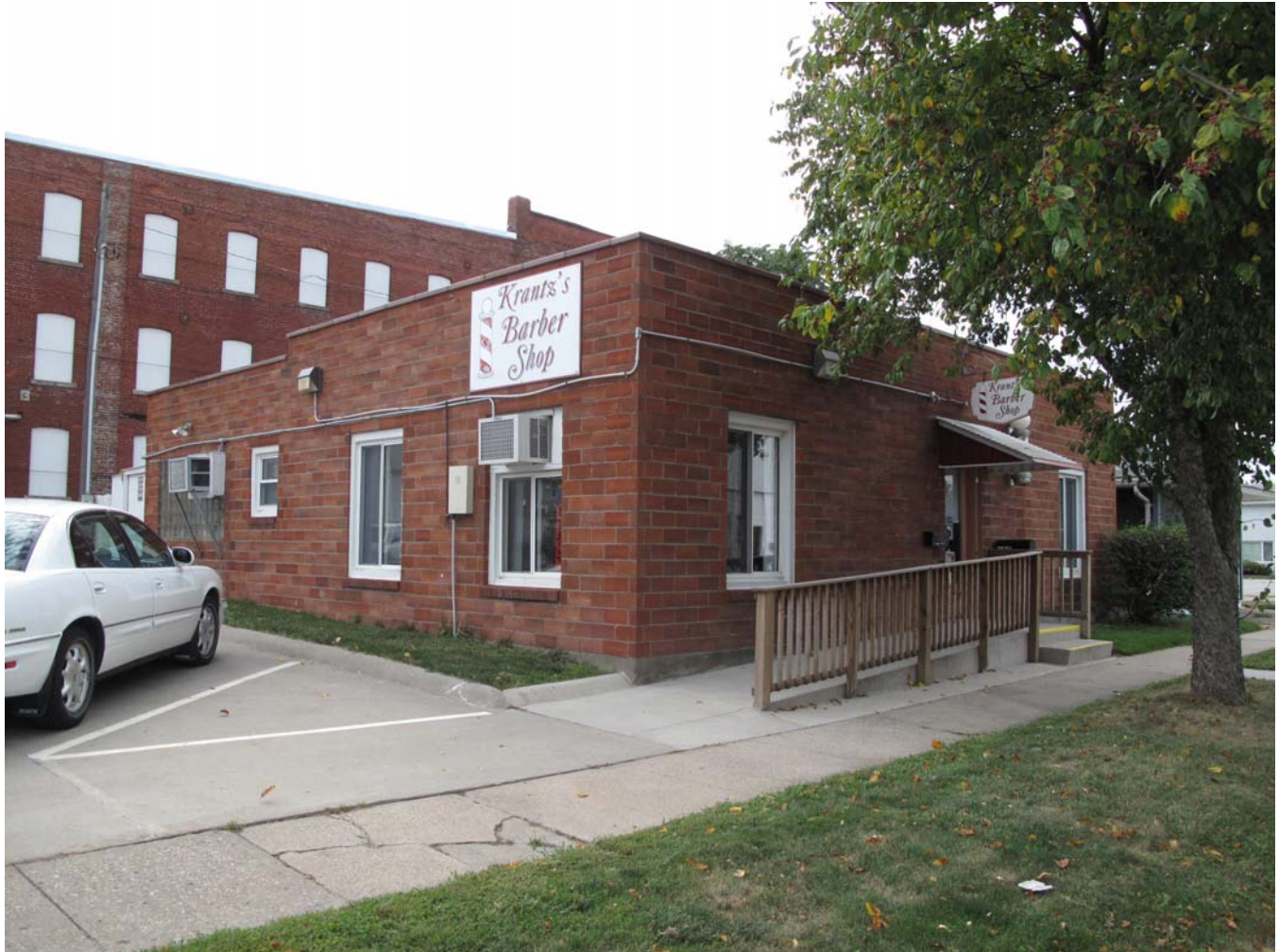
92-00588-002 - East and north elevations, looking southwest (McCarley, September 20, 2011)
