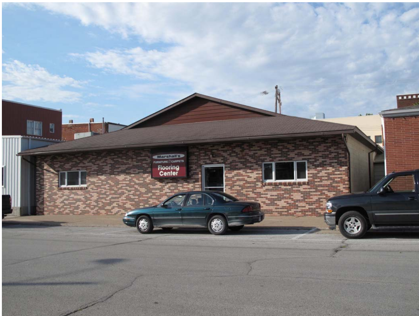
Photograph 92-00526-001 - South elevation, looking north (McCarley, September 20, 2011)
