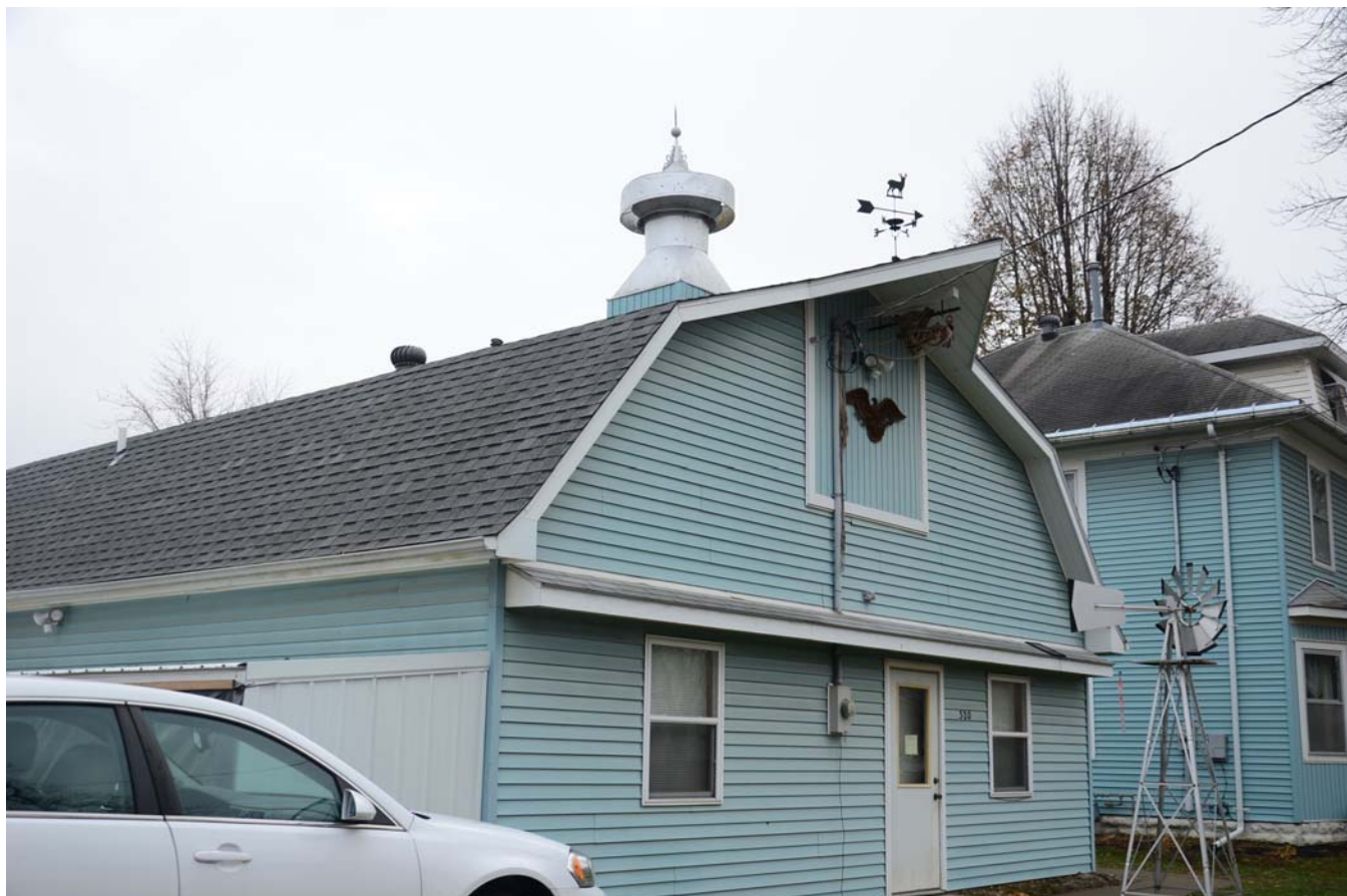
Photograph 92-00807-004 - Garage, looking southeast (December 2014)
