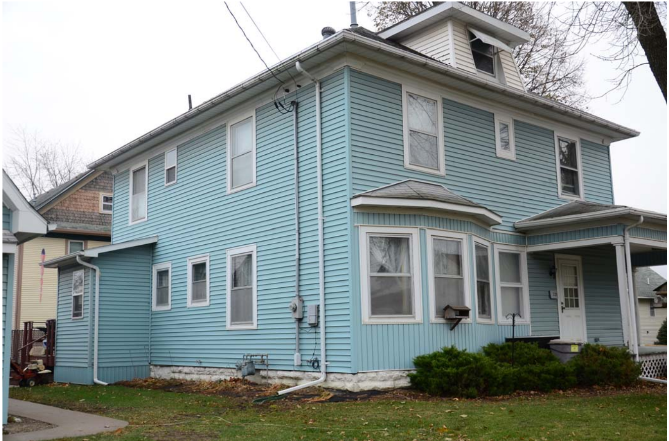
Photograph 92-00807-003 - House, looking southeast (December 2014)
