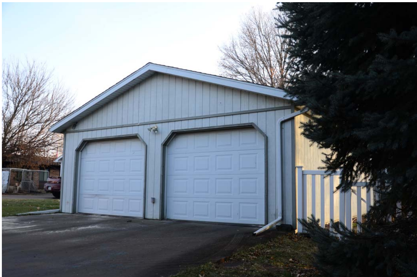
Photograph 92-00415-004 - Garage, looking northwest (December 2014)
