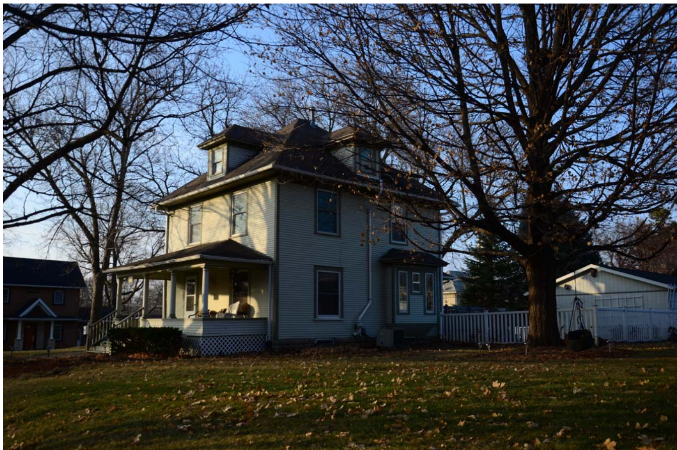
Photograph 92-00415-002 - House, looking northwest (December 2014)
