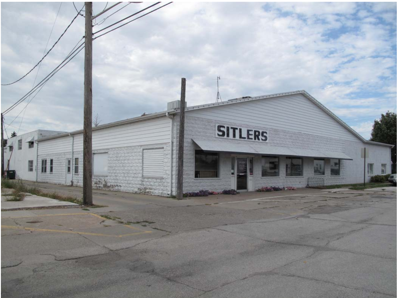
Photograph 92-00506-001 - South and east elevations of original building, looking northwest (McCarley, September 20, 2011)
