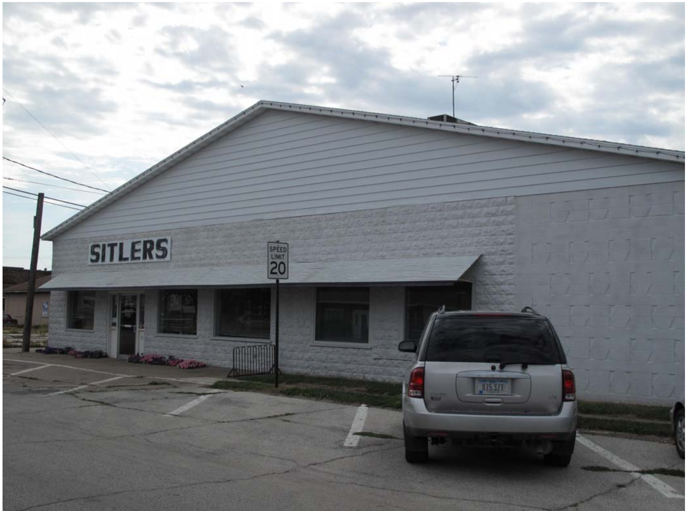
Photograph 92-00506-002 - East elevations of original building and north side addition with combined gable roof, looking southwest (McCarley, September 20, 2011)
