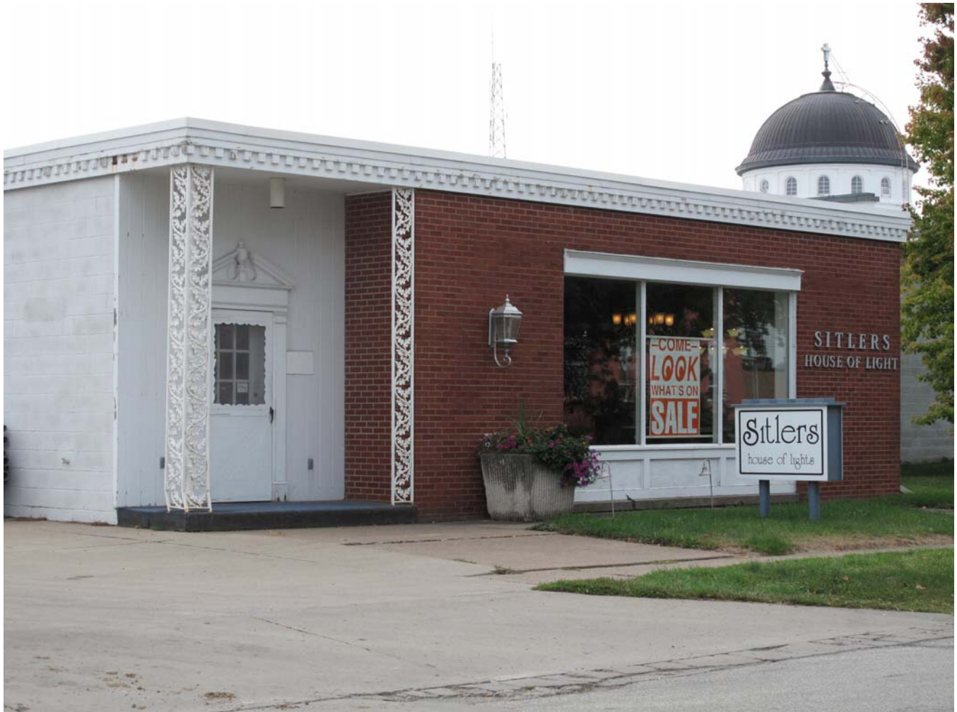
Photograph 92-00506-004 - North elevation of 1962 showroom addition, looking southwest (McCarley, September 20, 2011)
