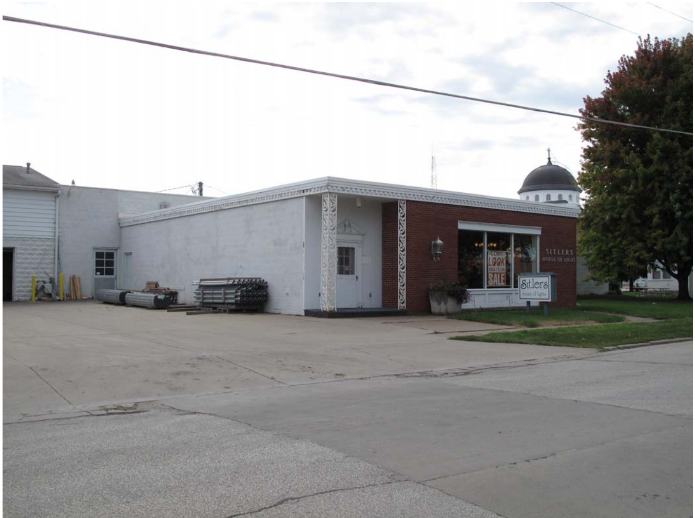
Photograph 92-00506-003 - East and north elevations of 1962 showroom addition, looking southwest (McCarley, September 20, 2011)
