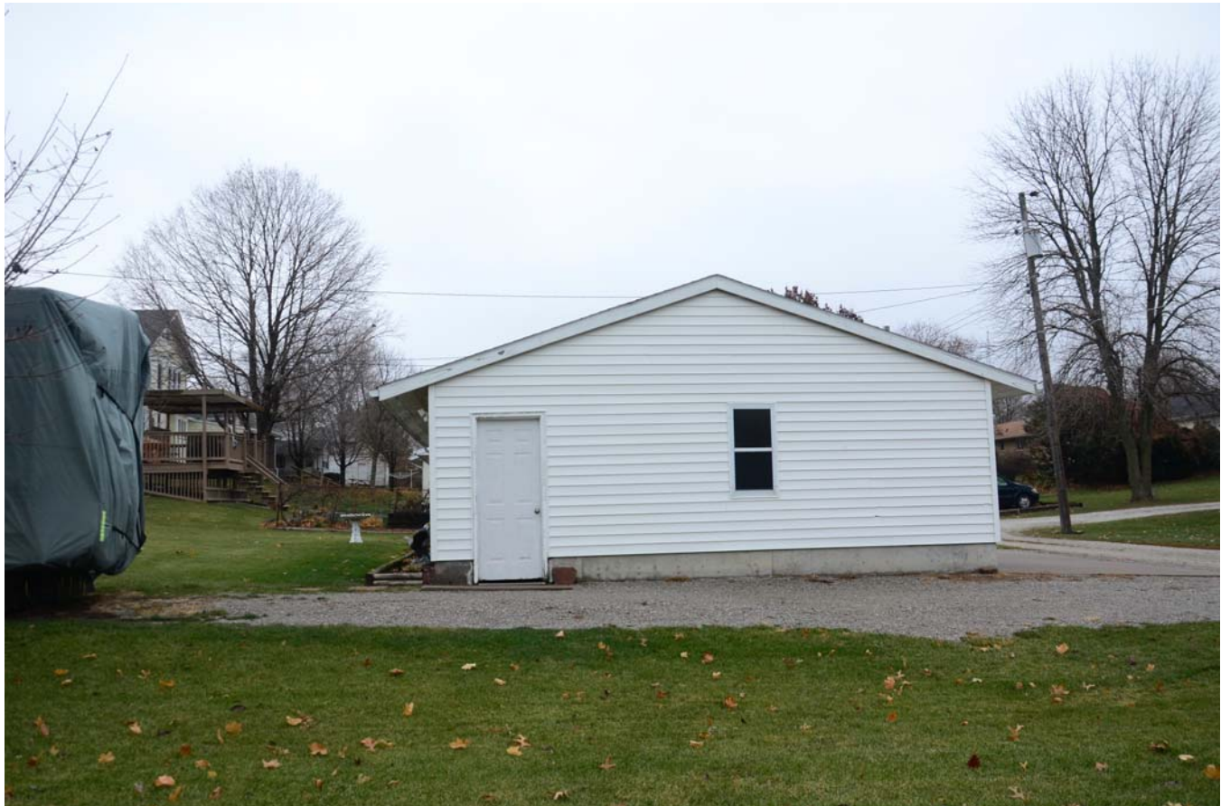
Photograph 92-00755-003 - Garage, looking east (December 2014)
