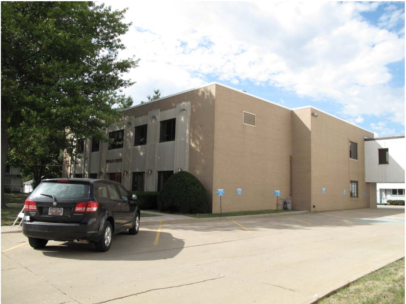
Photograph 92-00584-002 - South and east elevations, looking northwest (McCarley, September 20, 2011)
