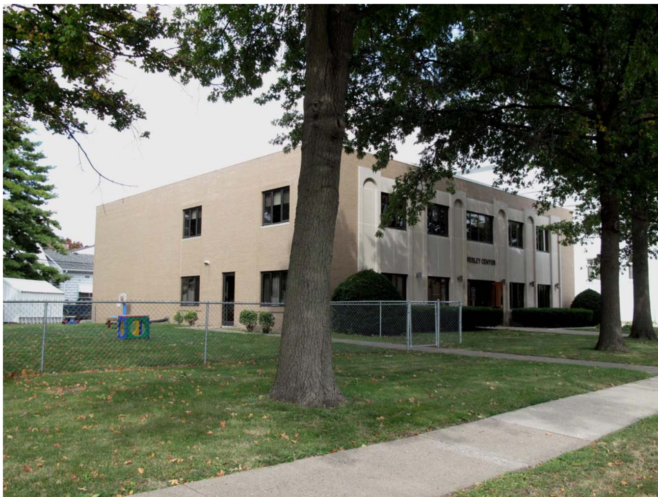
Photograph 92-00584-001 - West and south elevations, looking northeast (McCarley, September 20, 2011)
