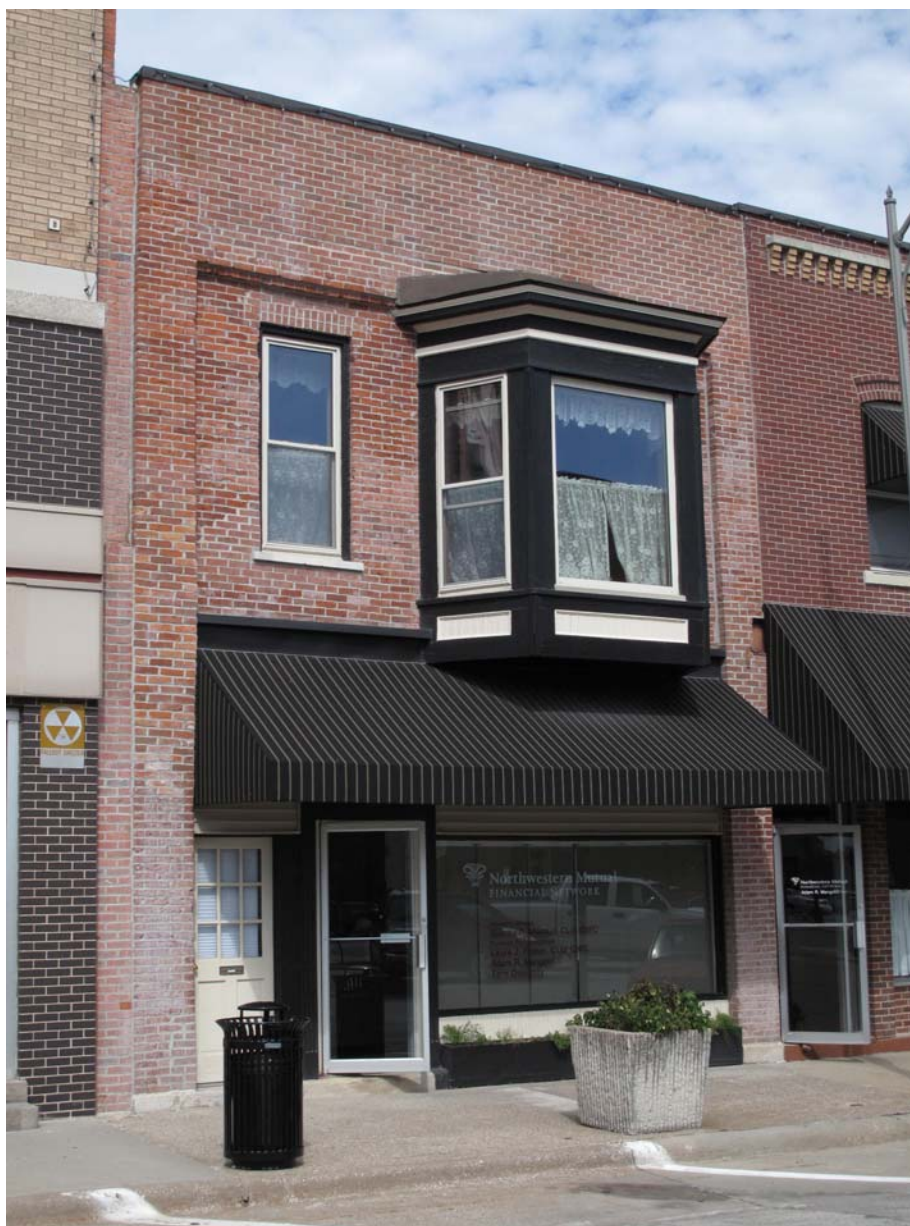
Photograph 92-00521-001 - South elevation, looking northeast (McCarley, September 20, 2011)
