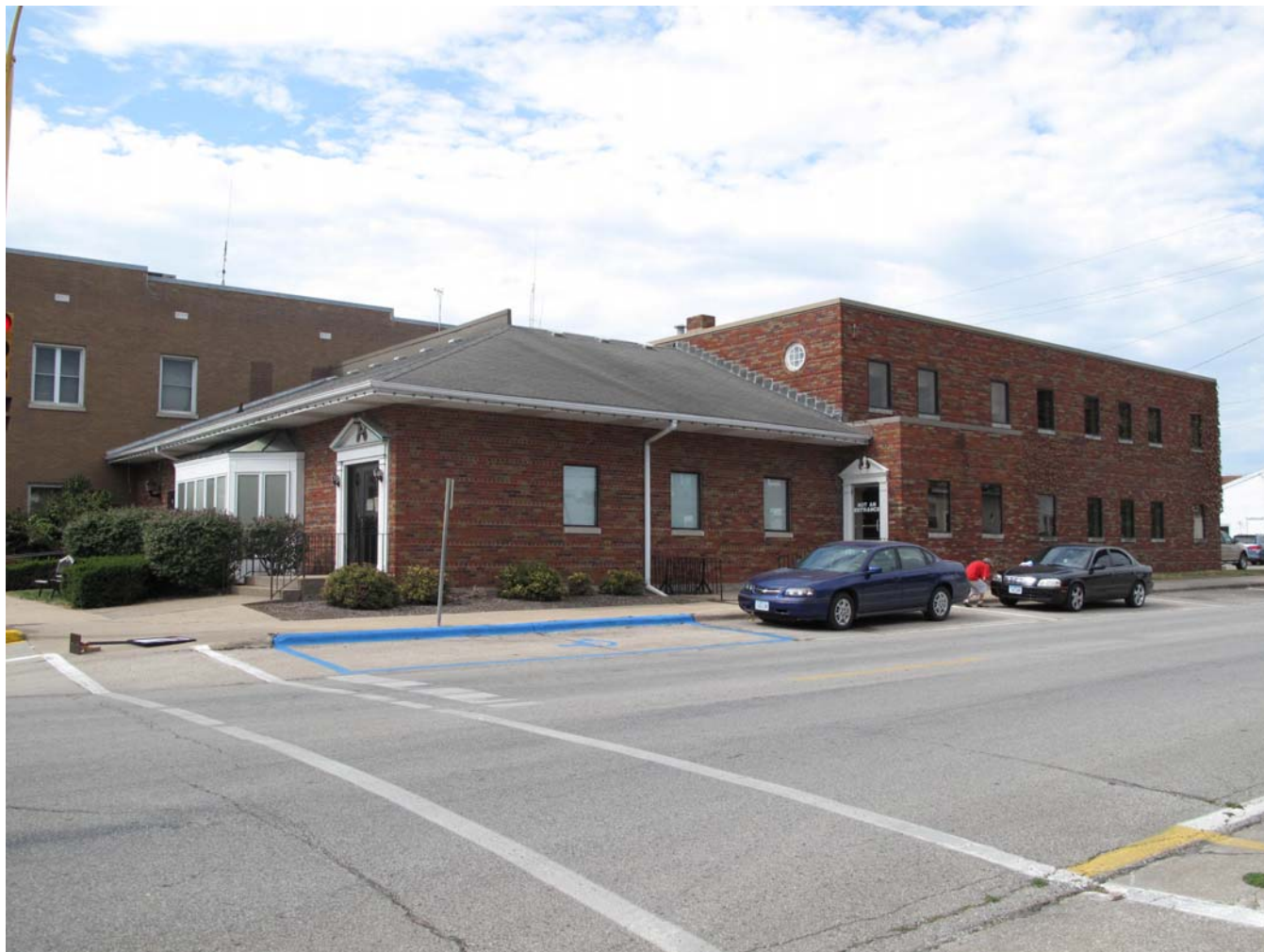
Photograph 92-00161-002 - South and east elevations, looking northwest (McCarley, September 20, 2011).
