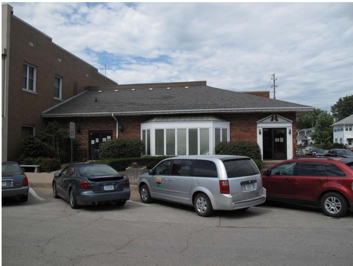
Photograph 92-00161-001 - South elevation, looking north (McCarley, September 20, 2011).
