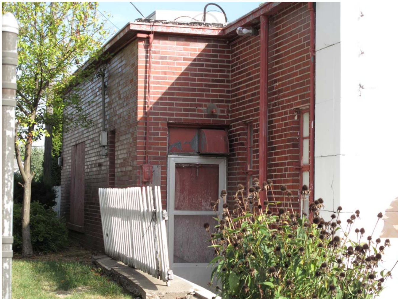
Photograph 92-00600-003 - North elevation, looking southeast (McCarley, September 20, 2011)
