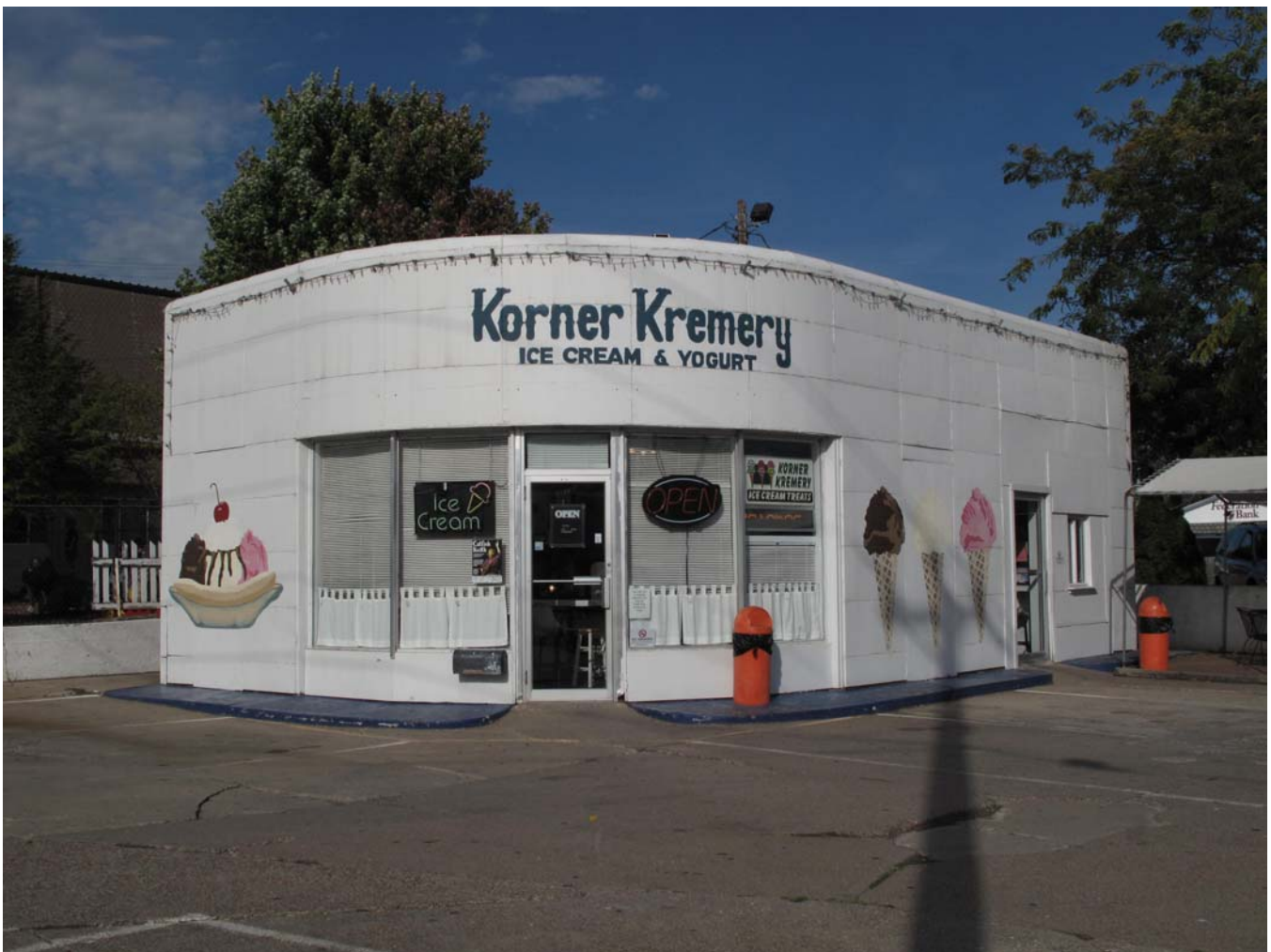
Photograph 92-00600-001 - West and south elevations, looking northeast (McCarley, September 20, 2011)
