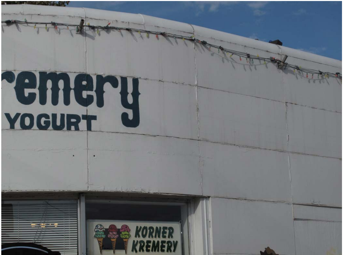
Photograph 92-00600-002 - Detail of wall, looking northeast (McCarley, September 20, 2011)
