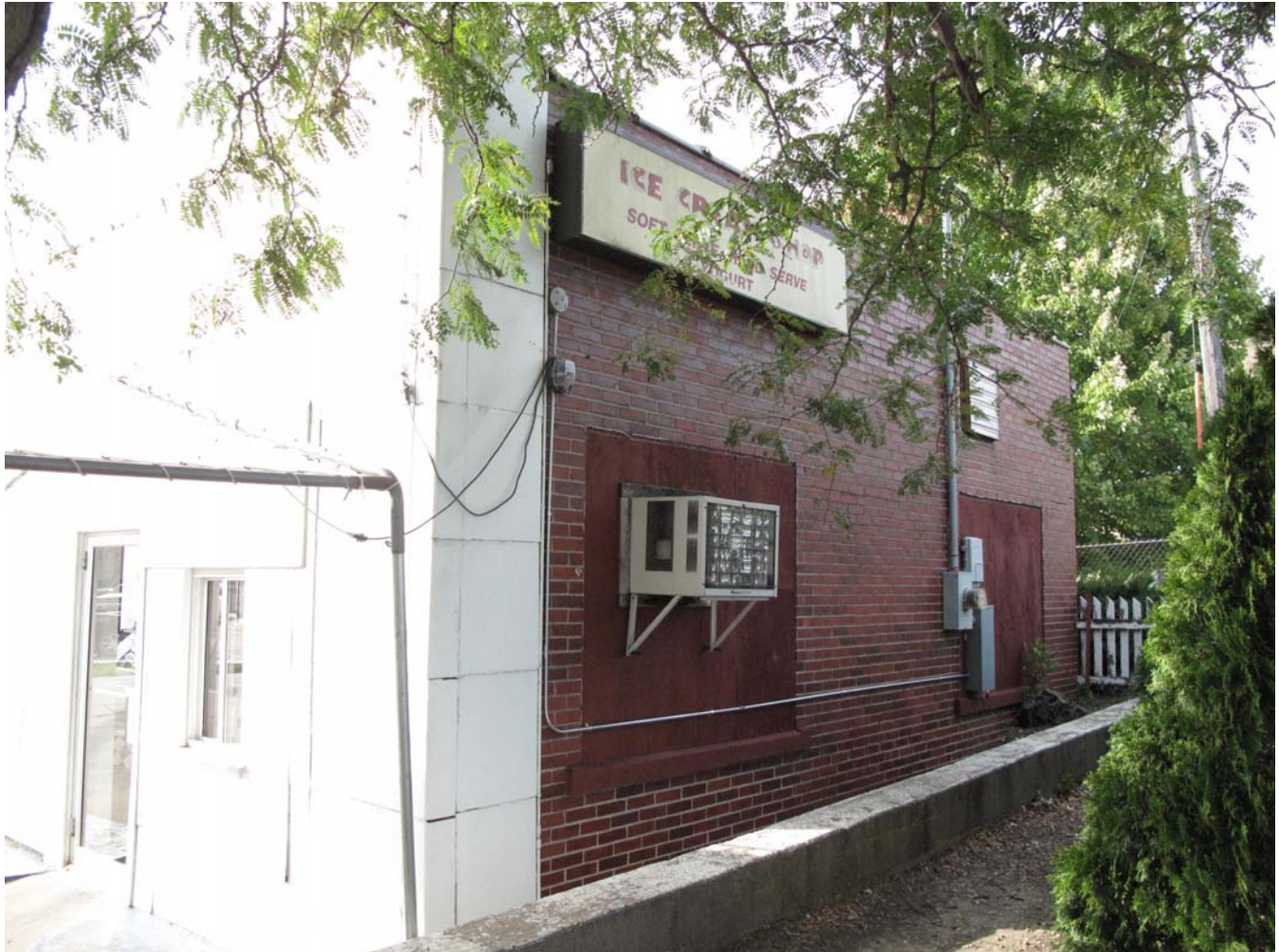
Photograph 92-00600-004 - East elevation, looking northwest (McCarley, September 20, 2011)
